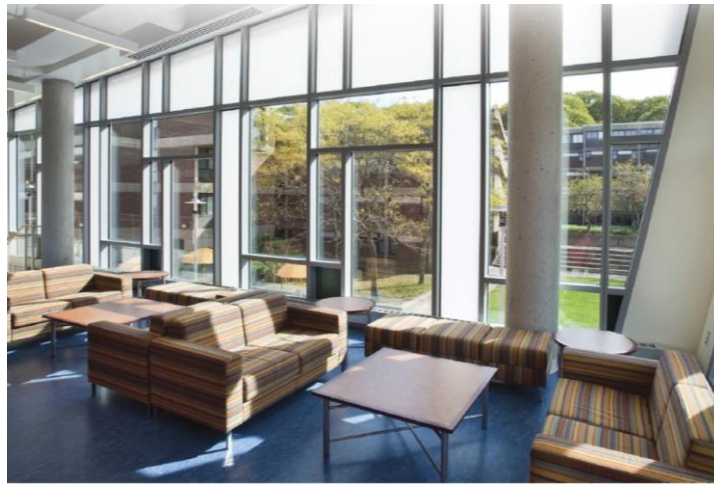
Figure 5: Granular filled aerogel windows: Nobel Halls at SUNY Stony Brook, NY, USA applied over large areas in new buildings for day lighting purposes (Berardi 2015)
