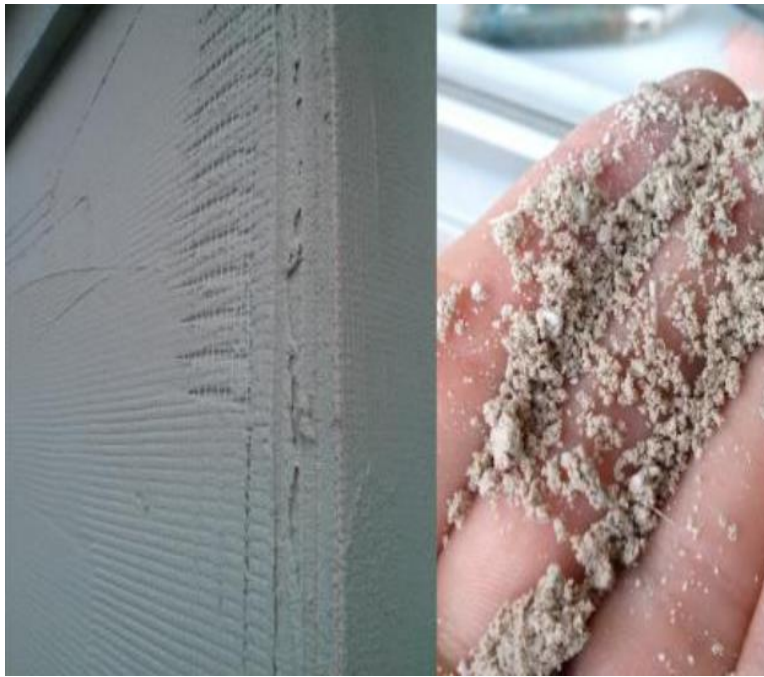
Figure 14: Applied reinforcement mesh (left), FIXIT 222 insulation plaster (right) (Proskurnina, n.d.)
