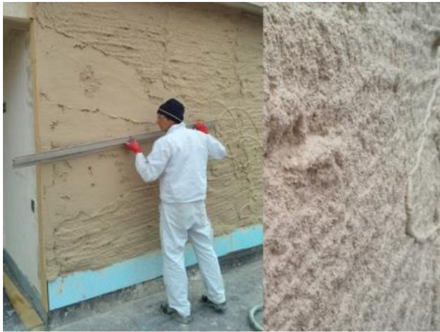
Figure 12: Levelling off FIXIT 222(left), surface of FIXIT 222(right) (Proskurnina, n.d.)
