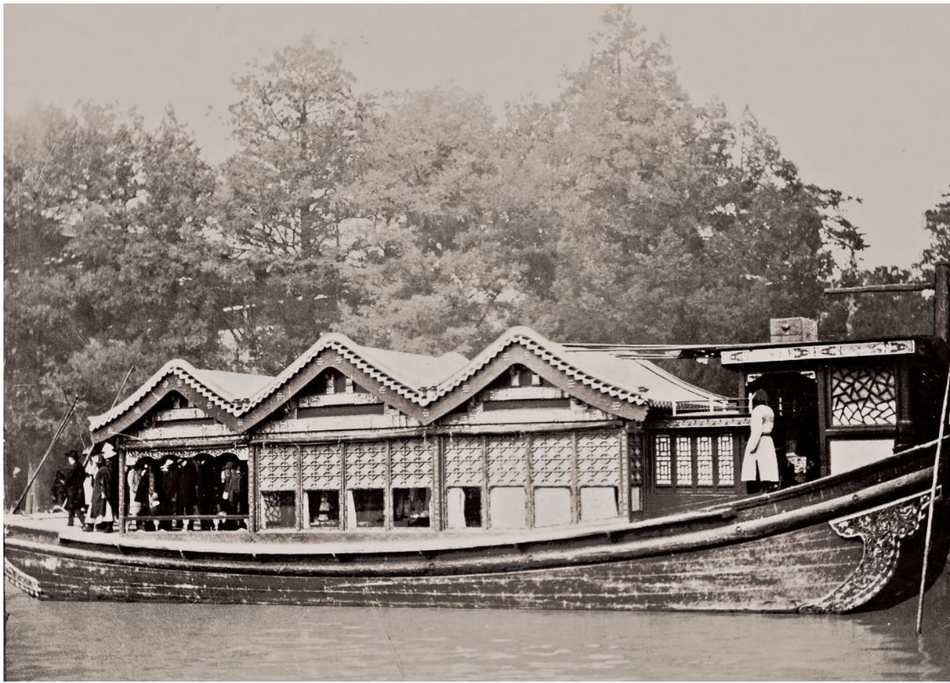
Fig. 4.3.2-3 An old photo of the Shuiyunxiang .
