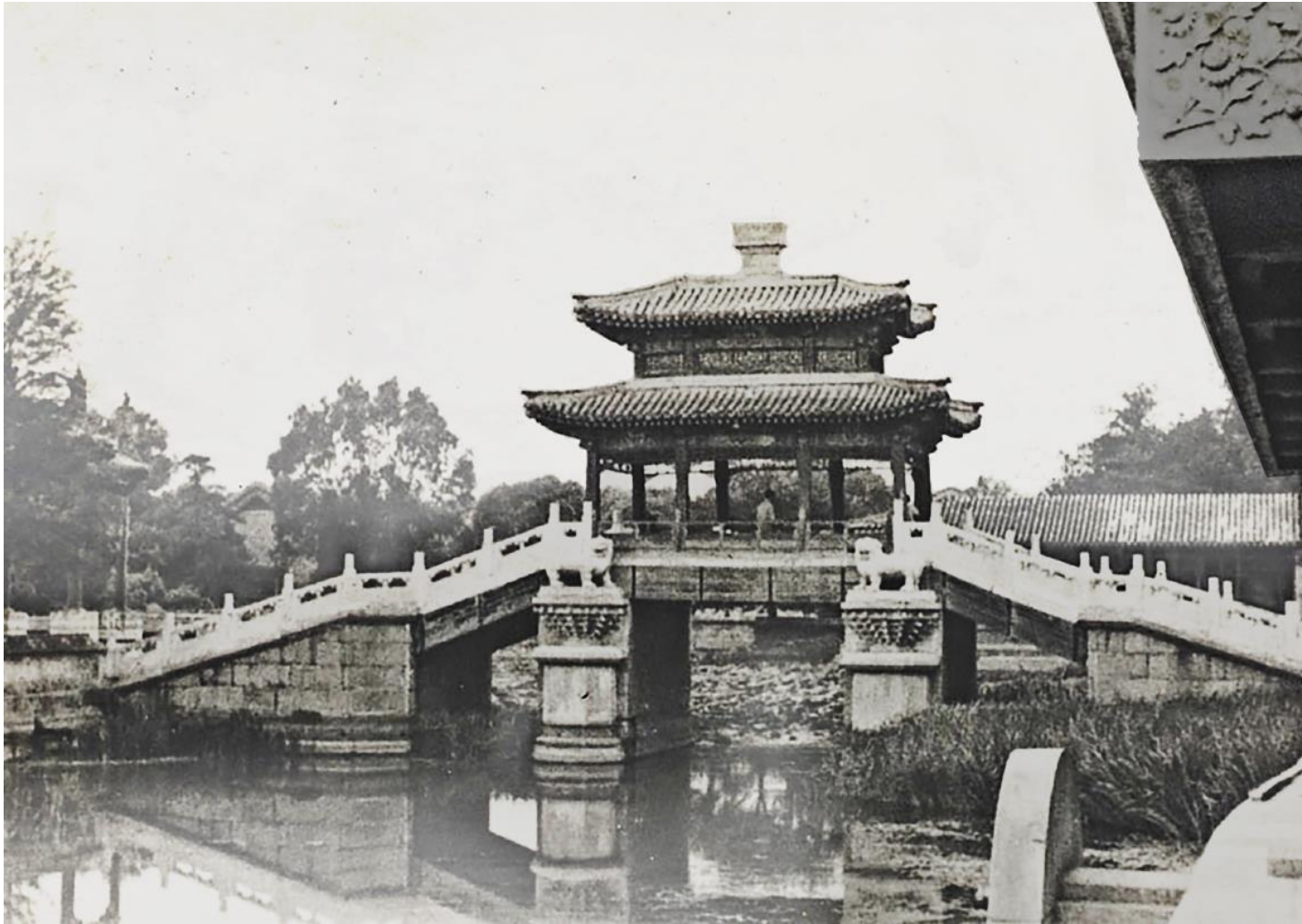
Fig. 3.3.3-11 Looking at the Xing Bridge on the Shi Fang.
