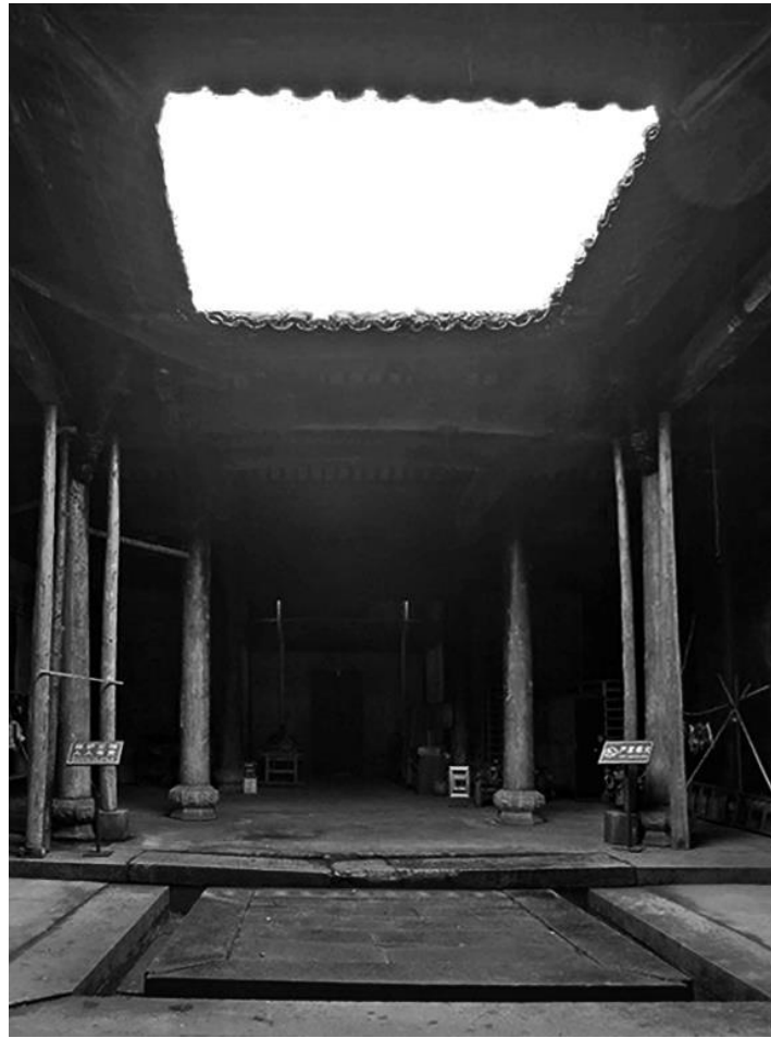
Fig. 4.1.1-11 The patio of the main hall unit of Yangchuan Wu.
