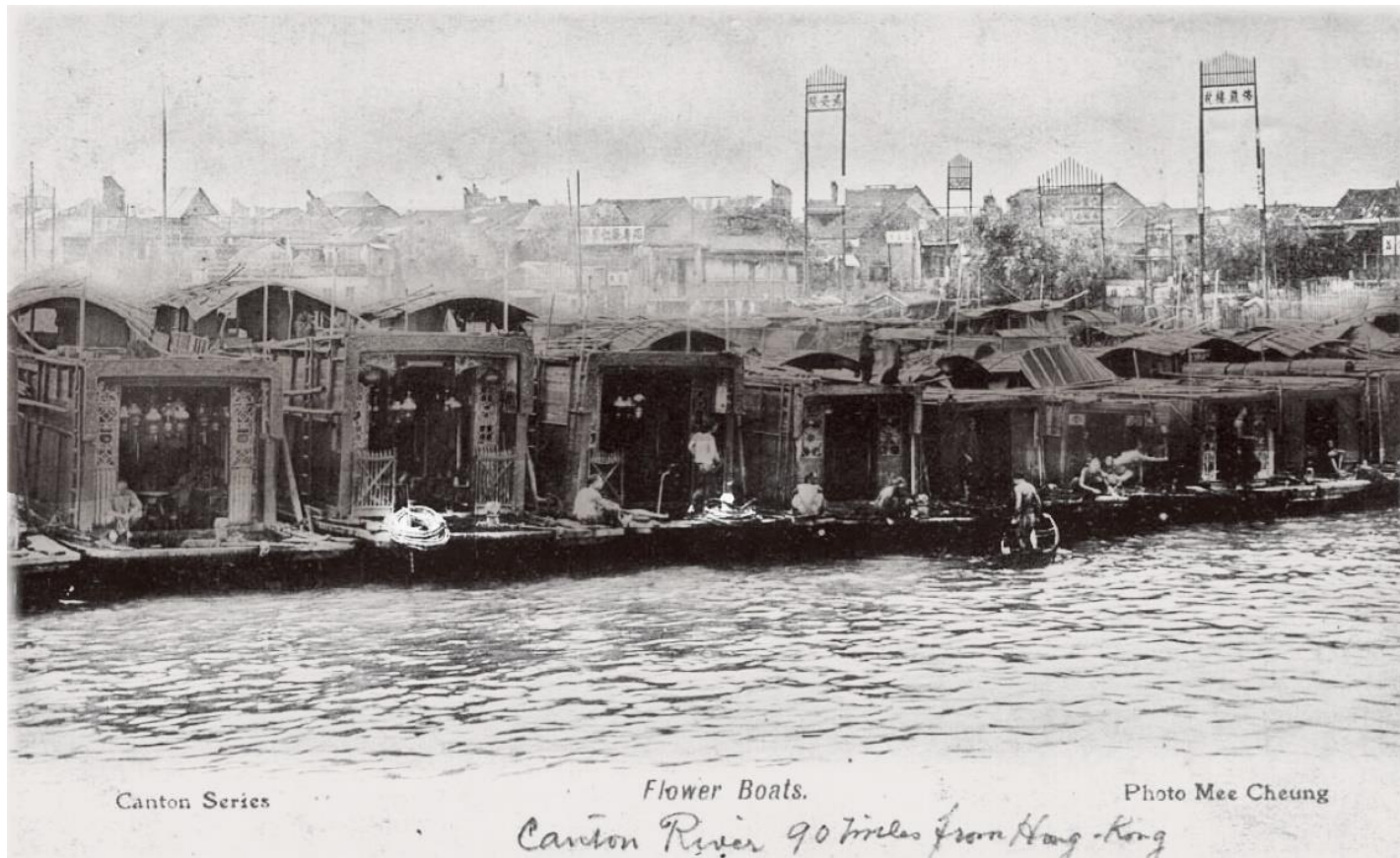
Fig. 2.4.2-16 The cables on the flower boats' decks.
