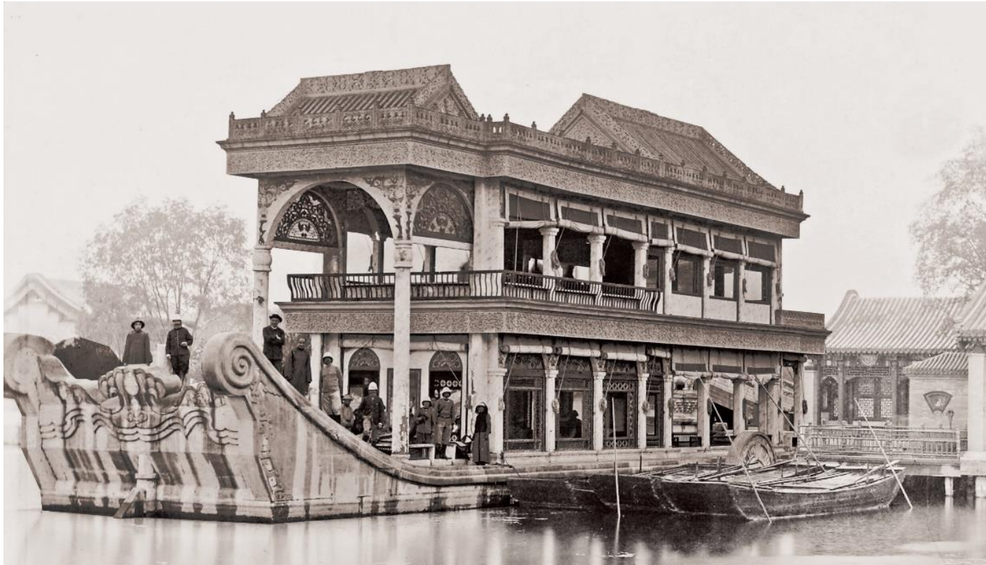
Fig. 3.3.3-15 The vintage photograph showcased the southern “front façade.”
