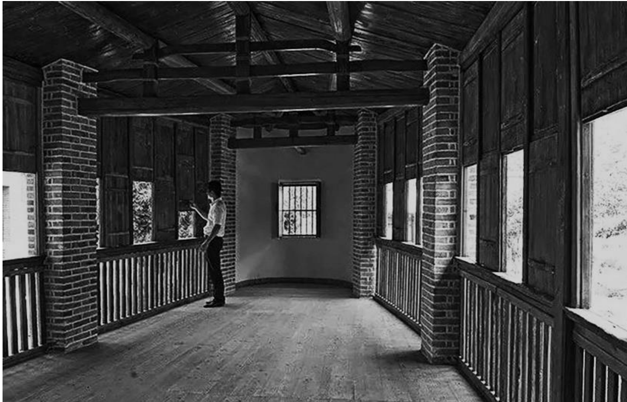
Fig. 4.3.4-9 Inner space of the upper floor.
