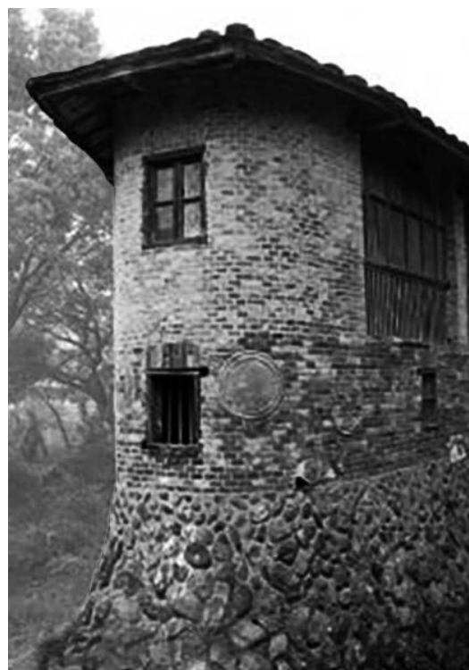
Fig. 4.3.4-3 The three-sided sloping roof. (left)
