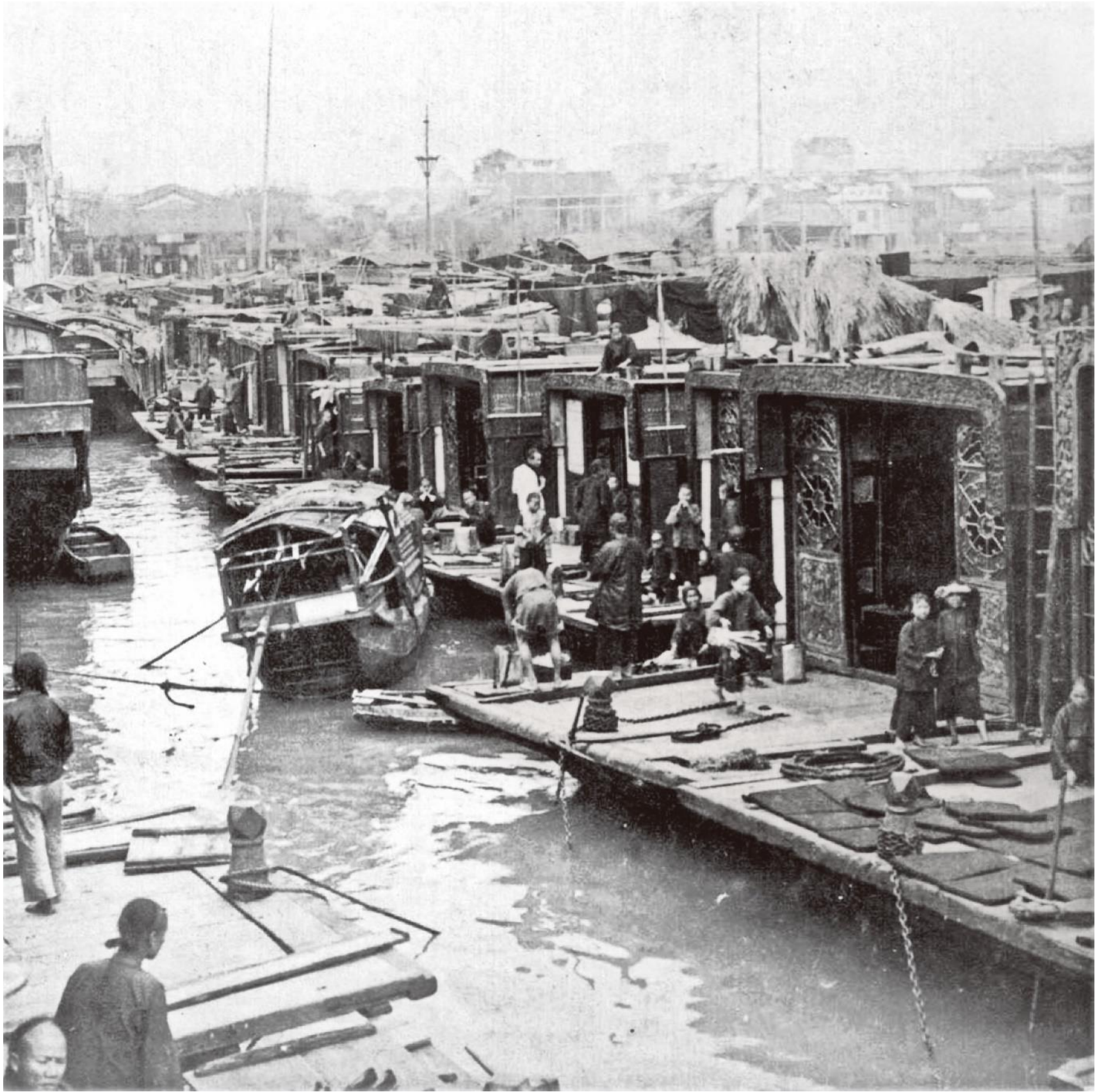
Fig. 2.4.2-9 The water street formed by the zidongting .
