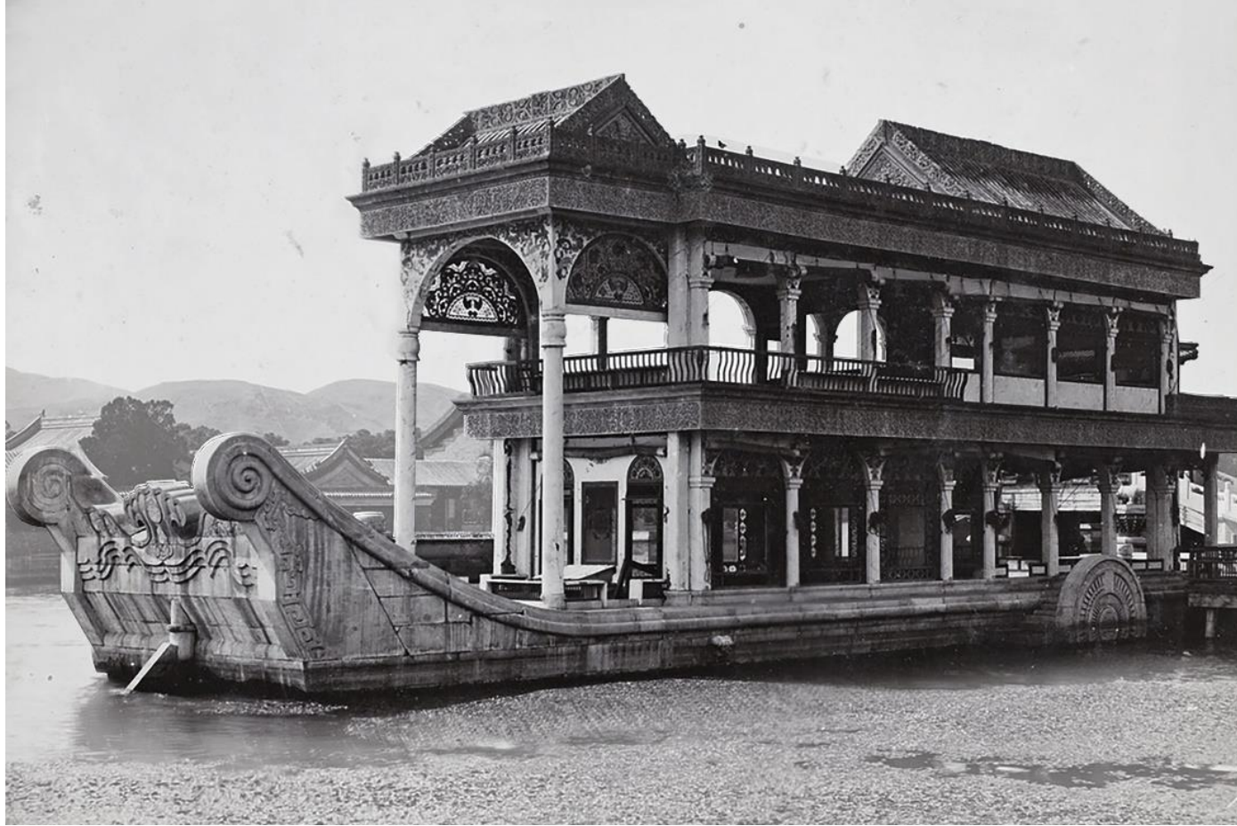
Fig. 3.3.3-5 The three parts of the roof.
