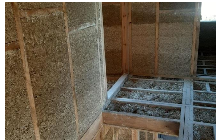
Fig. 69. Hemp insulation technology - Hempire Mix
