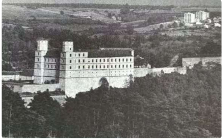
[88] Willibaldsburg Castle on top of the hill and in the background the first apartment buildings (Seidlkreuz).
