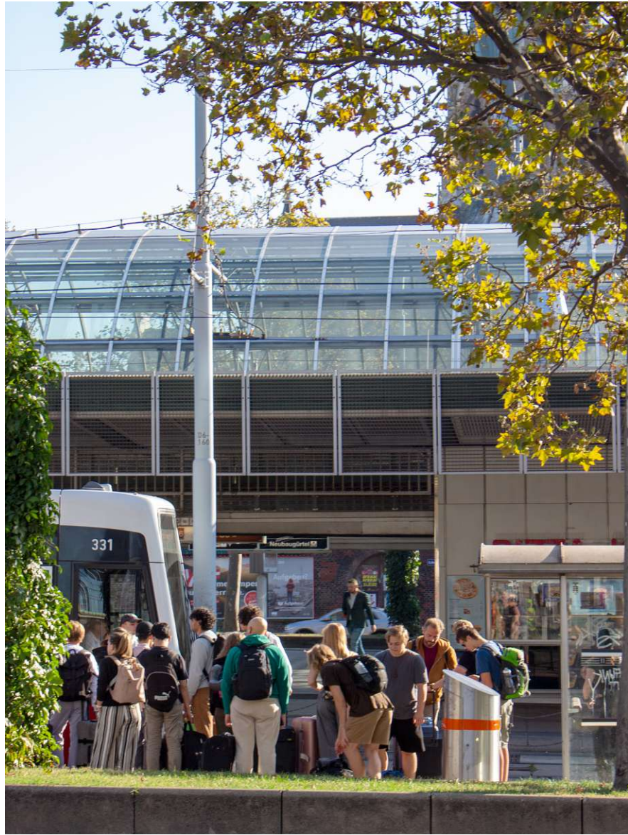
Figure 71: Tram Station Westbahnhof
