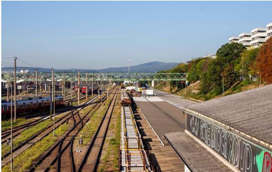
Figure 78: Westbahn and Rustensteg
