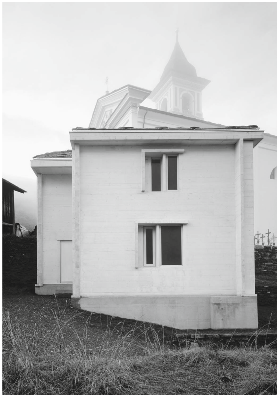
Abb. 56 Totenstube in Vrin, Gion A. Caminada, 2002
