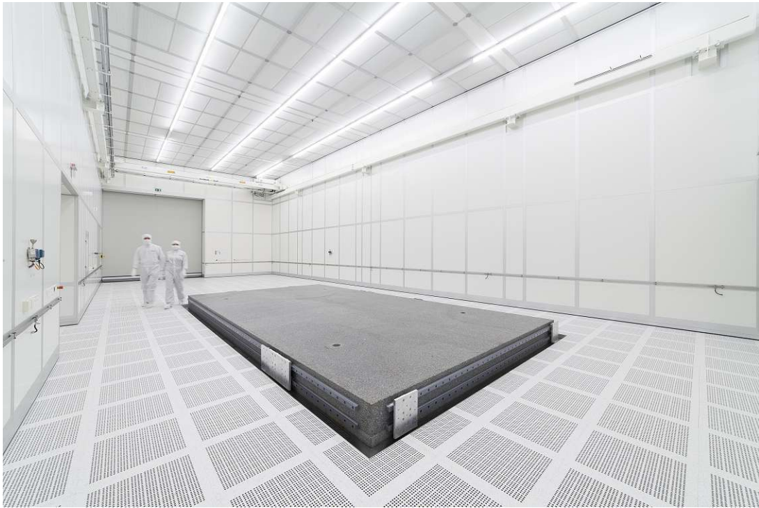
Abb. 2.2: View into the ISO 5 clean room at OHB. Note the holes in the floor to enable downward facing laminar flow. Also note the worn garment and the granite block for optical measurements to minimise contamination and changes in temperature.
