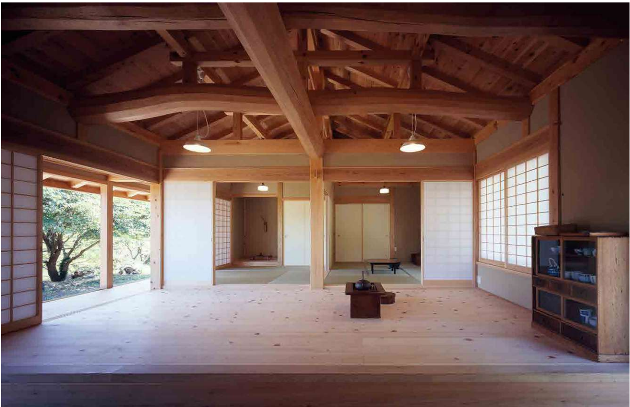
Fig. 20 - traditional Japanese timber frame construction
