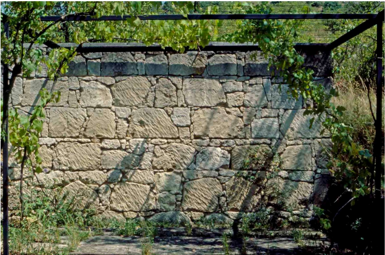
Fig. 98 - calcareous sandstone walls from St. Margarethen quarry
