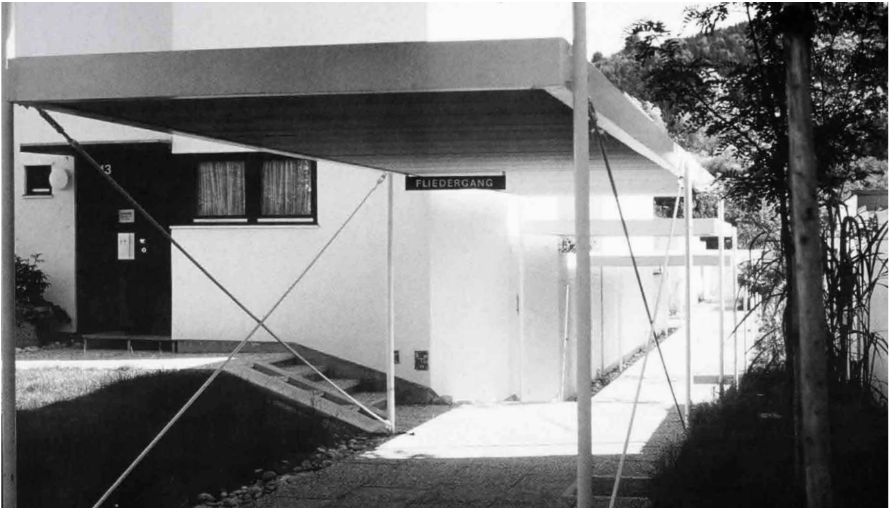
Fig. 87 - Puchenau II, 1992 - steel structure sheltering pedestrian routes
