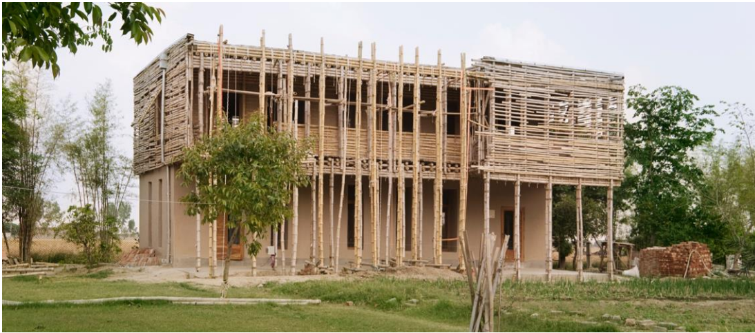
Abbildung 70: Schulgebäude in Jar Maulwi (Quelle: Roswag-Ziegert, 2014, https://www.holcimfoundation.org/projects/locally-manufactured-cob-and-bamboo-school-building-jar-maulwi )
