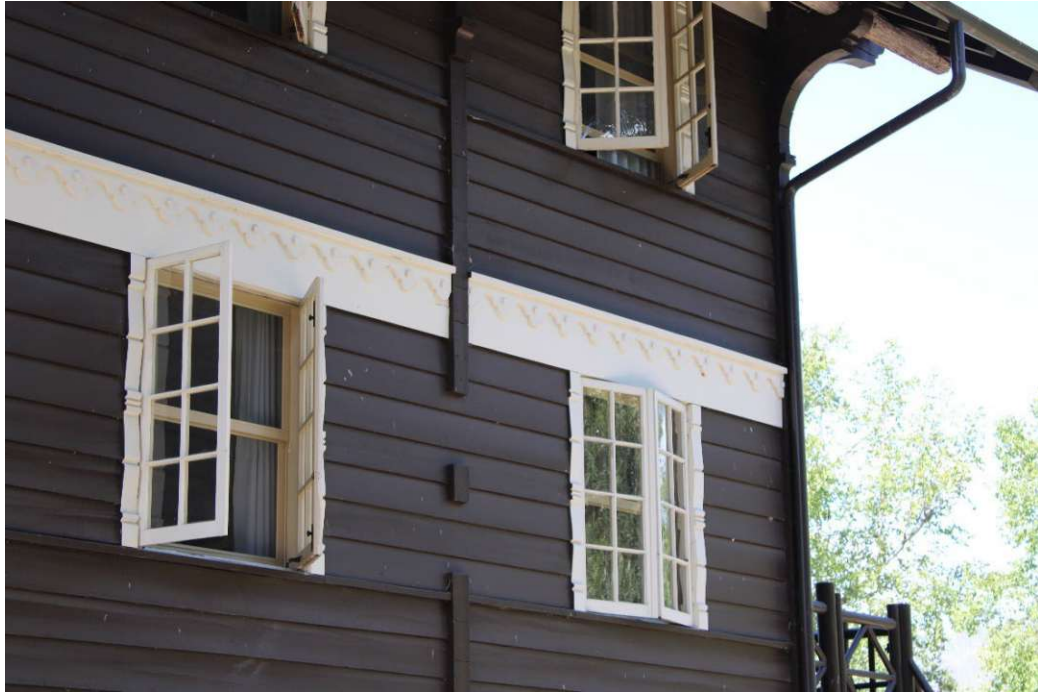
Fig. 44: North facade of Lake McDonald Lodge with the apparent protruding logs of interior walls
