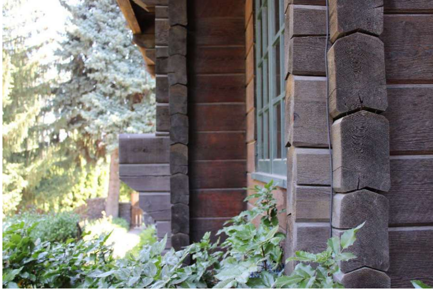
Fig. 21: Example of false V-notched log ends at the Koerner House in Spokane
