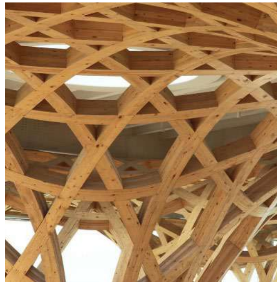
Abbildung 22: Dachtragwerk des Golfclubhauses in Yeosu, Shigeru Ban Architect 75
