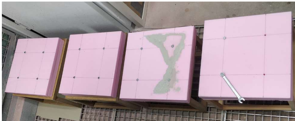
5.10 Cast formwork with the dowel guides viewed from above.
