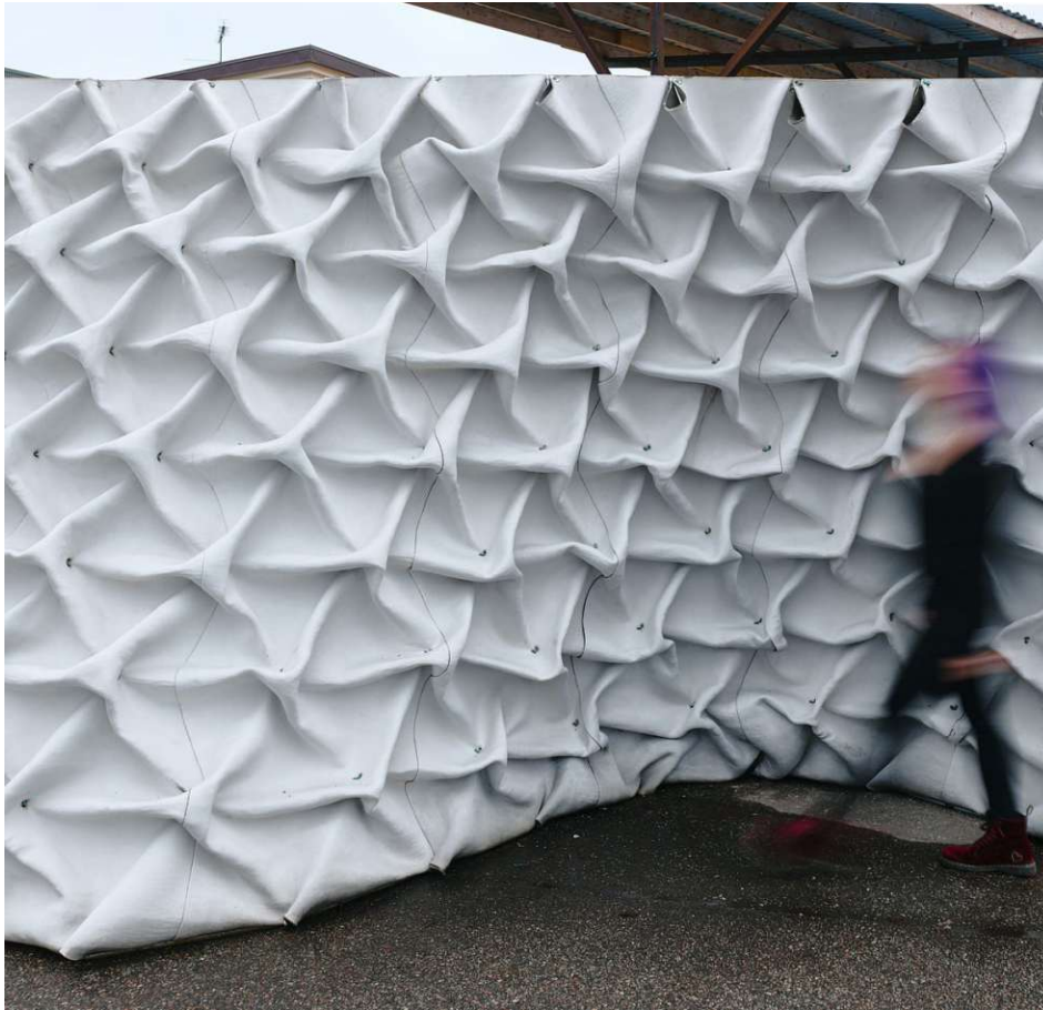
2.5 Concrete wall fabricated by smocking fabric. Prototype by Annie Locke Scherer Photo by Fredric Boukari
