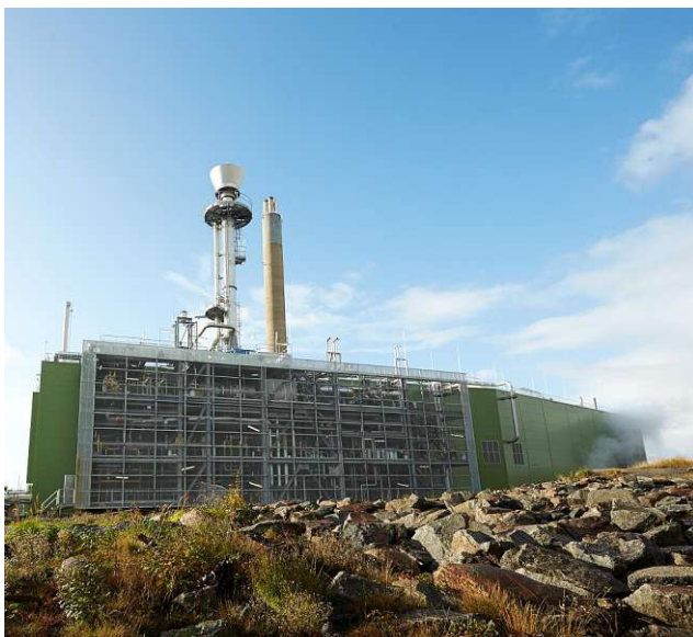
(a) GoBiGas plant Gothenburg
