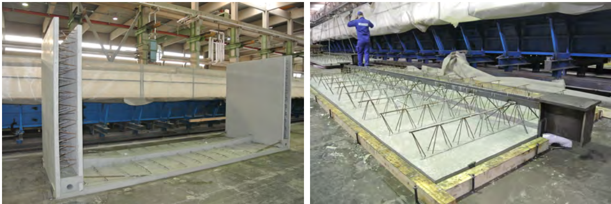
Fig. 6.4: Finished u-shaped cross-section and deck slab with stabilizing beam on casting table
