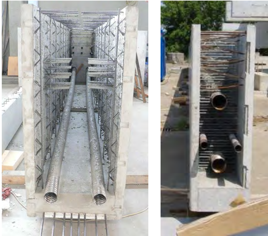
Fig. 2.2: Cross-sections of the designed lightweight thin-walled precast girders with the girder made of lattice-girder floor slabs on the left and the girder made of double wall elements on the right (Wimmer (2016))
