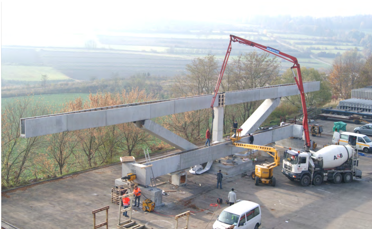
Fig. 2.3: Large-scale experiment on girder out of lattice-girder slabs - Filling of the girder with cast in-situ concrete
