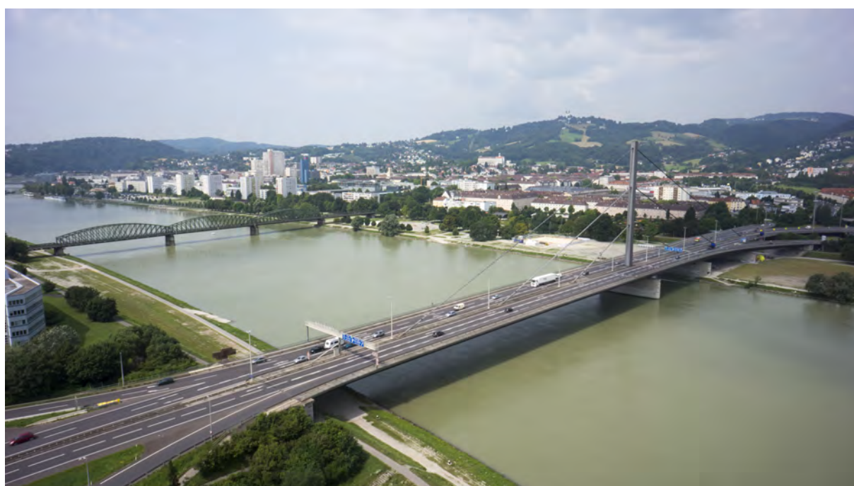
Fig. 7.2: The original Voest bridge from 1973 (ASFINAG, 2013)
