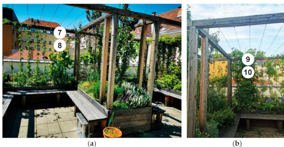
Figure 8. Images of the installed sensors at the green pergola at Schuhmeierplatz School: (a) position of the temperature and humidity sensors on the left side of the pergola; (b) position of the temperature and humidity sensors on the right side of the pergola.
