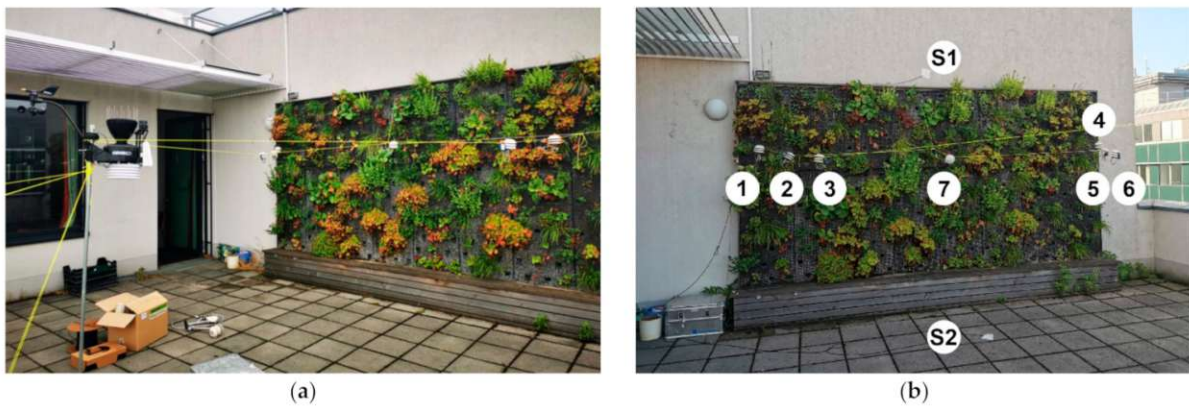
Figure 3. Images of the installation of the sensors at Diefenbachgasse School: (a) position of the weather station; (b) position of the temperature and humidity as well as surface temperature sensors.
