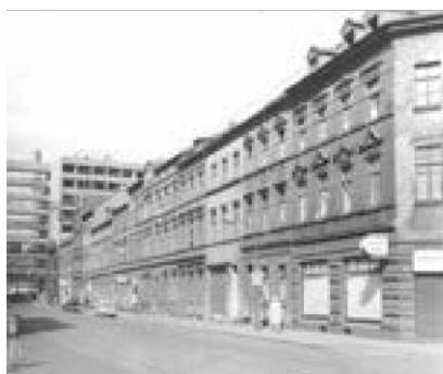
Fig. 74: 4. Werthausen Strasse (residential buildings demolished)
