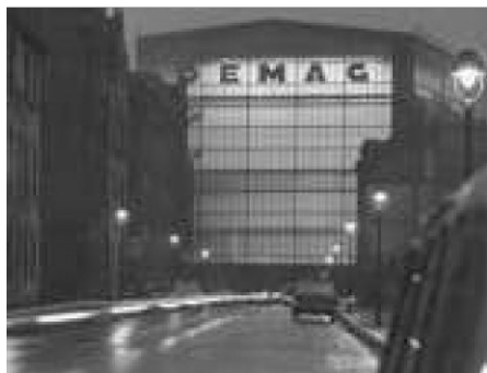
Fig. 77: 7. Sedanstrasse (residential buildings demolished)
