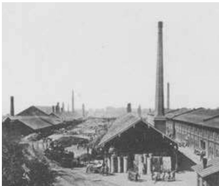
Fig. 62: H. J. Vuygen & Co. - Production of Fireproof Stones at Wörthstrasse (1890)
