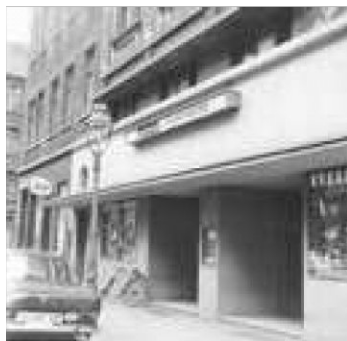
Fig. 78: 8. "Astoria Filmtheater" (demolished)
