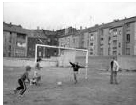
Fig. 79: 9. Courtyard before demolition (1976)
