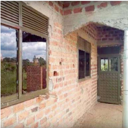
fig.17 Installed doors and windows.
