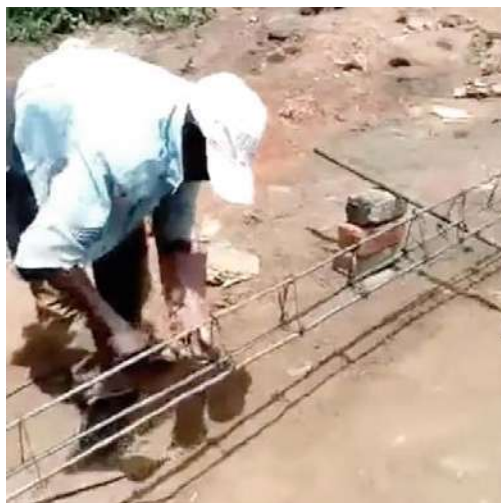
fig.11 Tying rebars.
