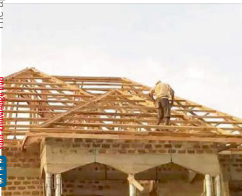
fig.13 Nailing the battens.
