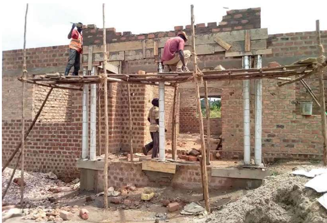
fig.10 Bricklayers on a makeshift scaffold.
