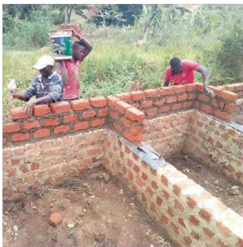
fig.9 Laying bricks for the walls.
