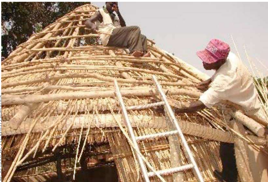
fig.12 Working on the suspended ceiling.
