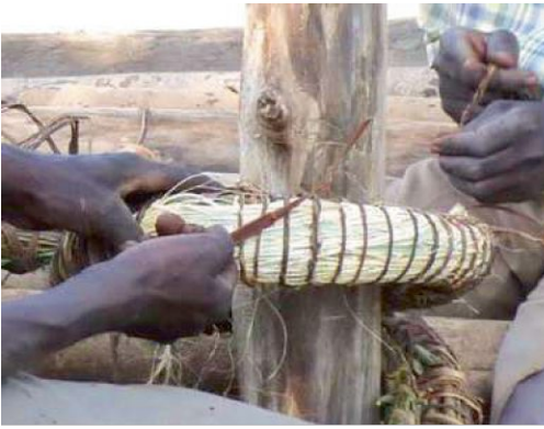
fig.8 Making the first ring around the center post.
