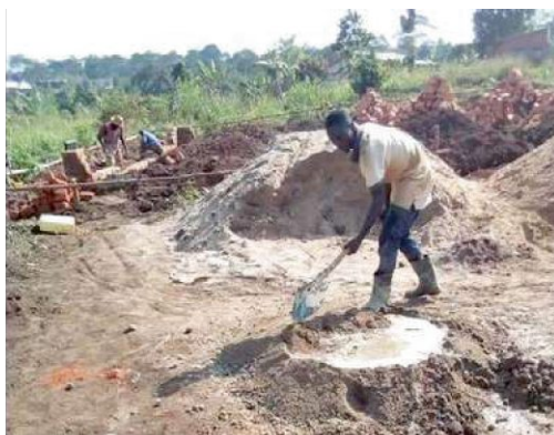
fig.8 Mixing cement mortar on the ground.
