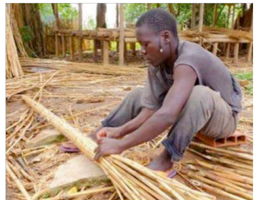
fig.11 Tying bundles of reed with sisal rope.
