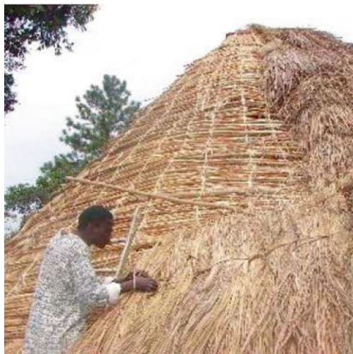
fig.14 Tying bundles of thatch.
