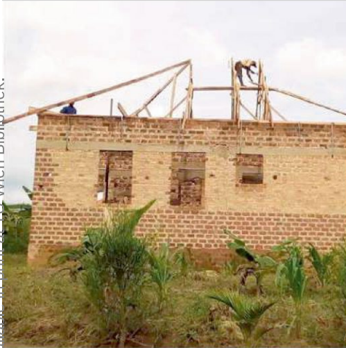
fig.12 Setting roof trusses and rafters.
