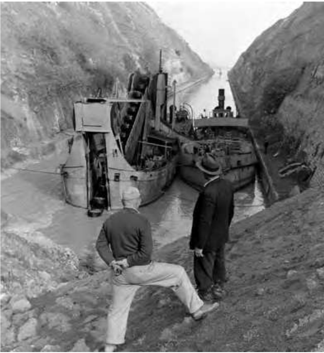
Figure 14: Transporting mud out of the canal
