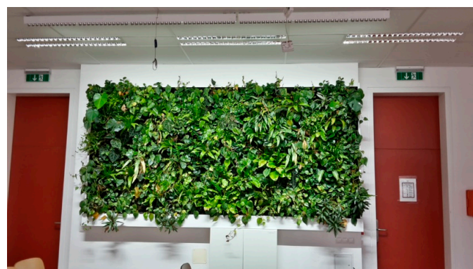
Figure 2. Fleece system in Building B.
