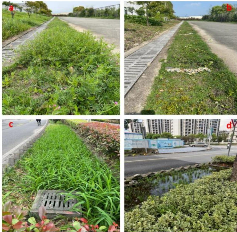
Figure 3: Swales (borrowed from Lu et al. 2023, 6)
