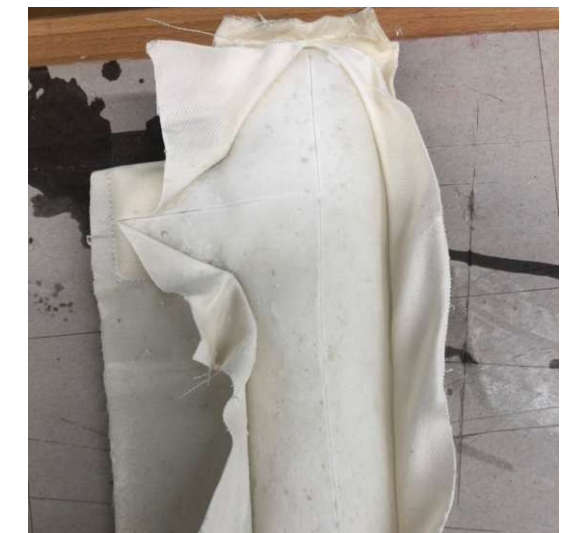
Fig.156. The white formwork was as if glued on the wax
