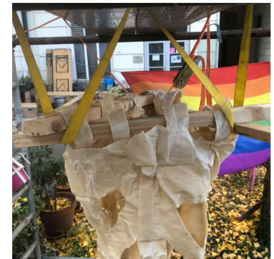
Fig.294. The suspension system of the formwork
