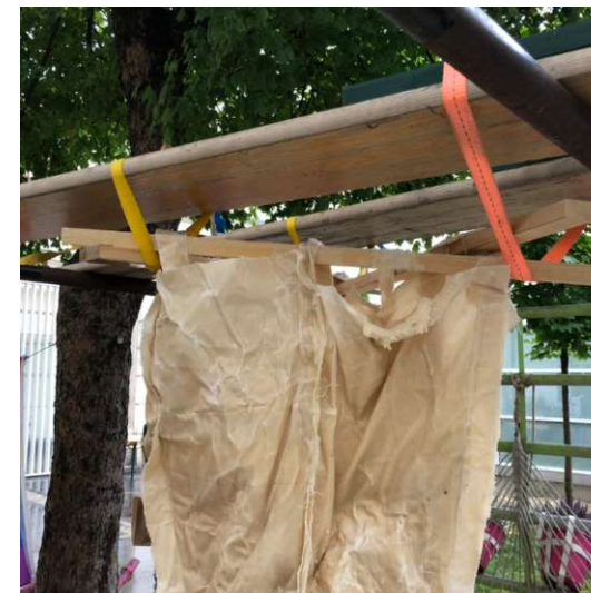
Fig.275. The suspension system of the formwork
