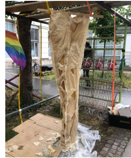
Fig.273. The suspended formwork, left side filled, right side empty
