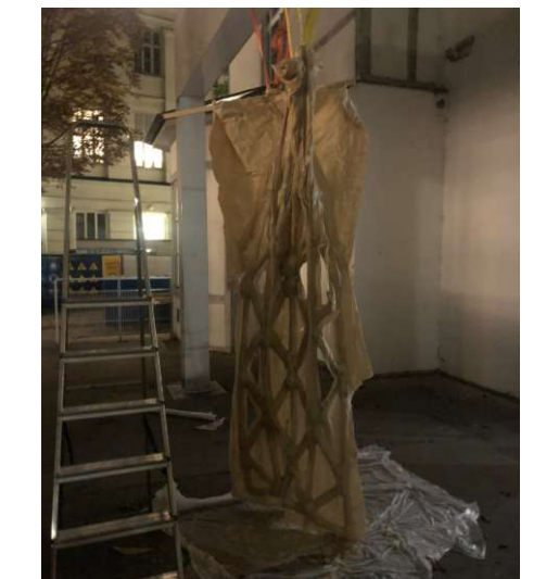
Fig.238. The structure half filled
