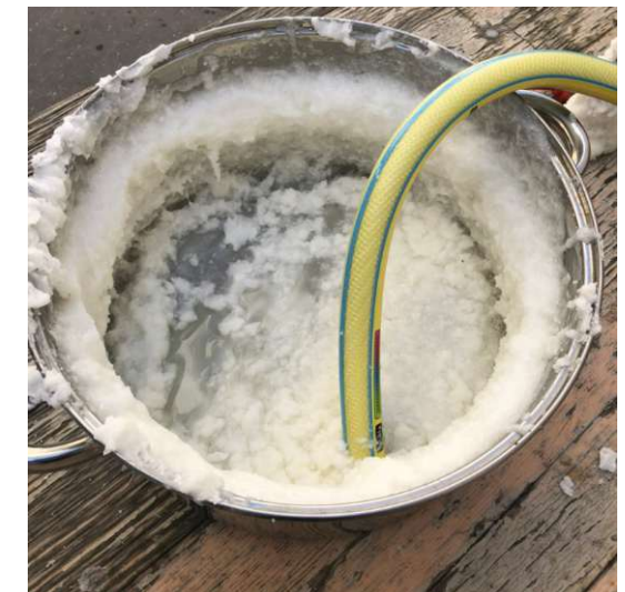
Fig.148. The formwork was filled using the injection moulding process
