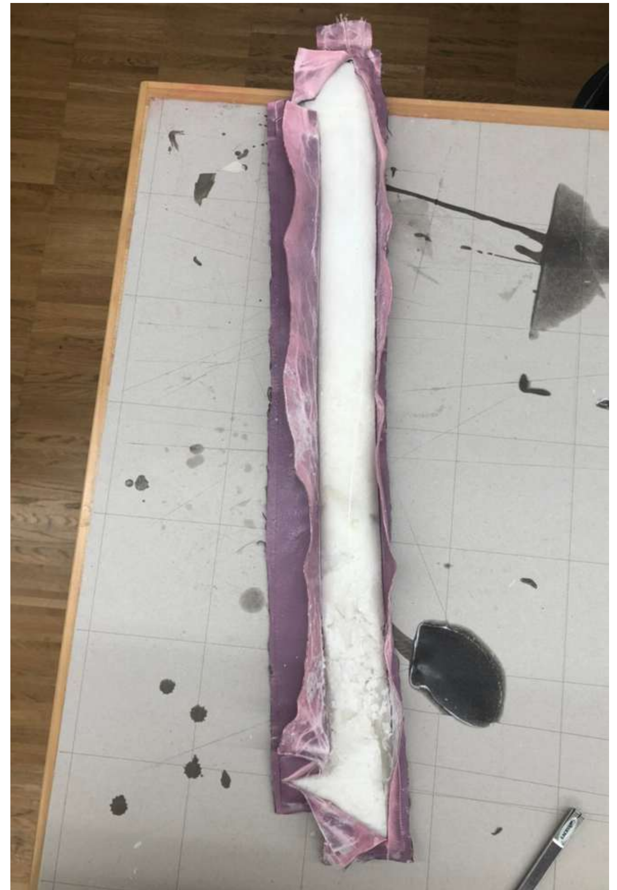
Fig.157. The injection moulding process produced many air bubbles in the formwork
