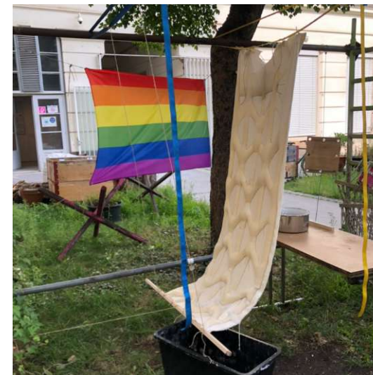
Fig.196. The filled formwork front
