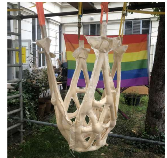
Fig.256. The filled formwork right
