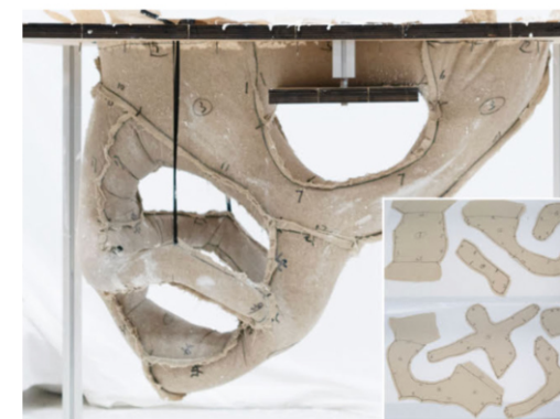
Fig.49. The realized and filled formwork
