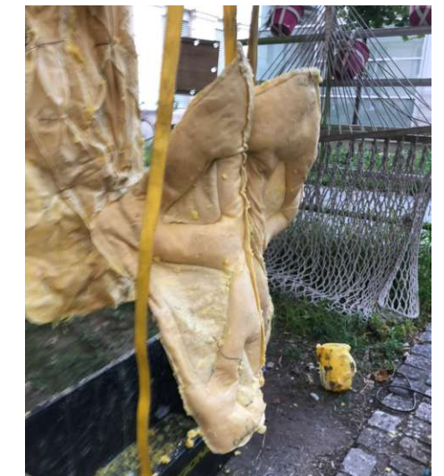
Fig.223. The formwork was hung from a scaffolding
