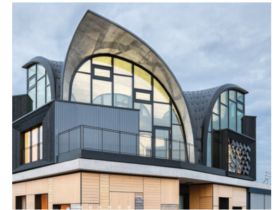
Fig.34. The built structure in Zurich
