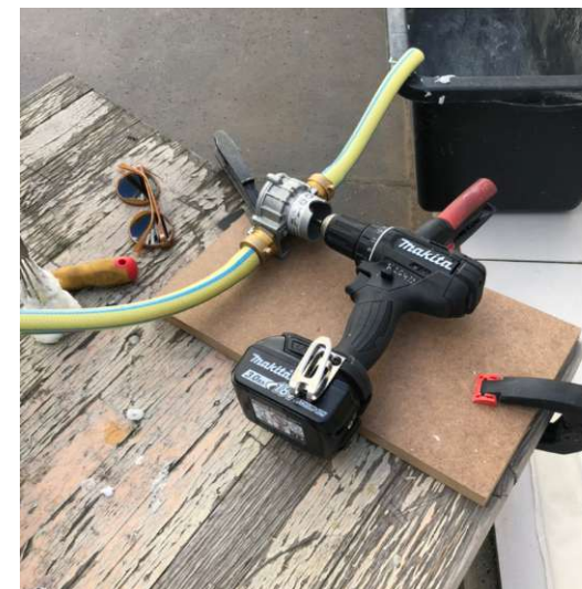
Fig.149. A drill pump was used to fill the formwork
