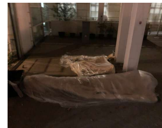
Fig.240. The structure was removed and placed on the ground
