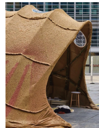
Fig.37. The substructure was made from bamboo
