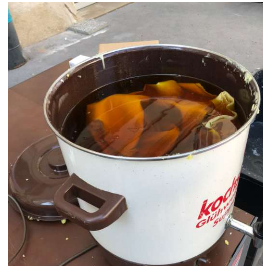
Fig.308. The formwork is soaked with wax
