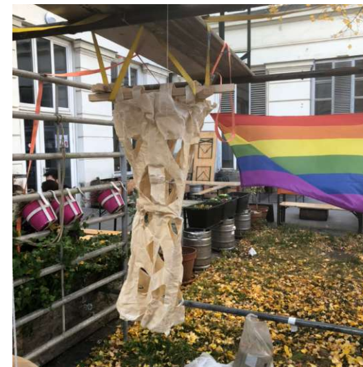
Fig.293. The formwork was hung from a scaffolding
