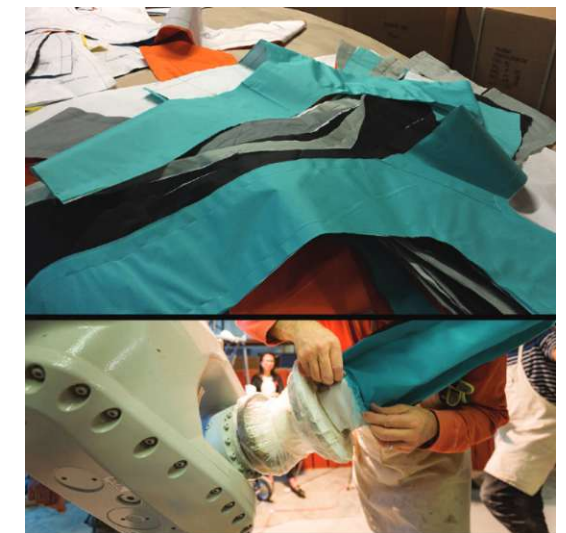
Fig.44. The sown formwork and its mounting on the robot
