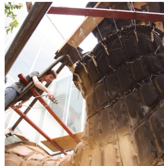
Fig.29. Tension connections & cable net structure
