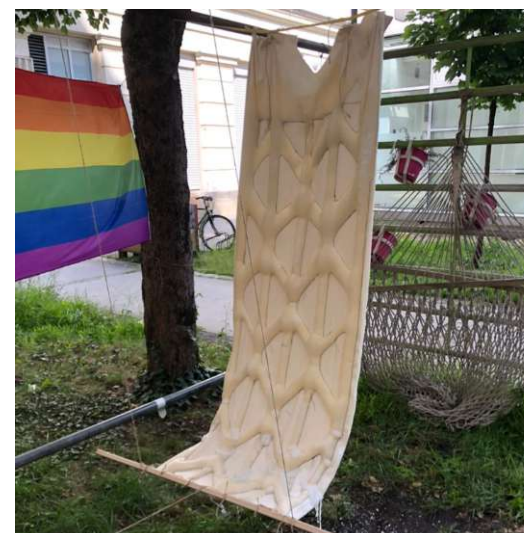
Fig.312. After casting the formwork is left hanging until solid
