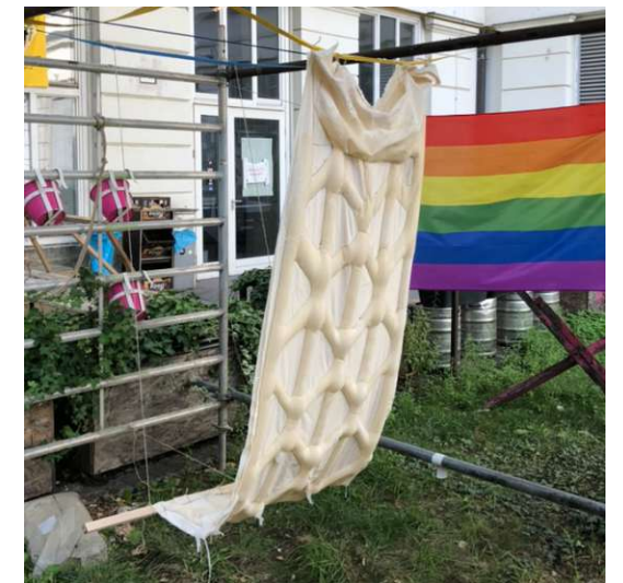
Fig.197. The filled formwork rearview
