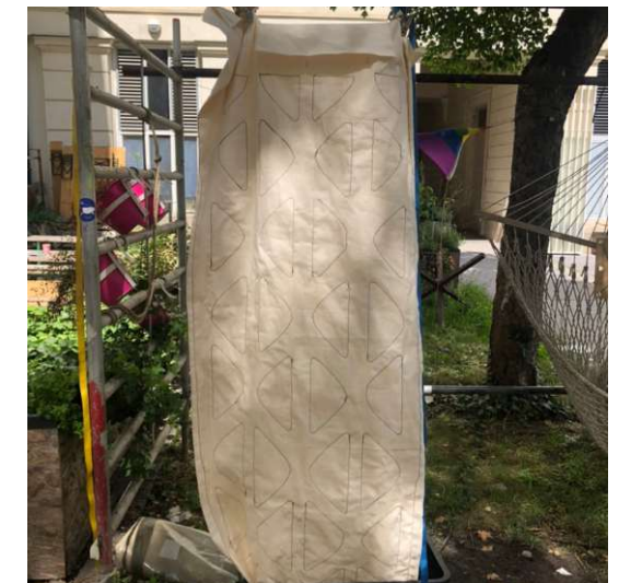
Fig.185. The formwork was hung from a scaffolding
