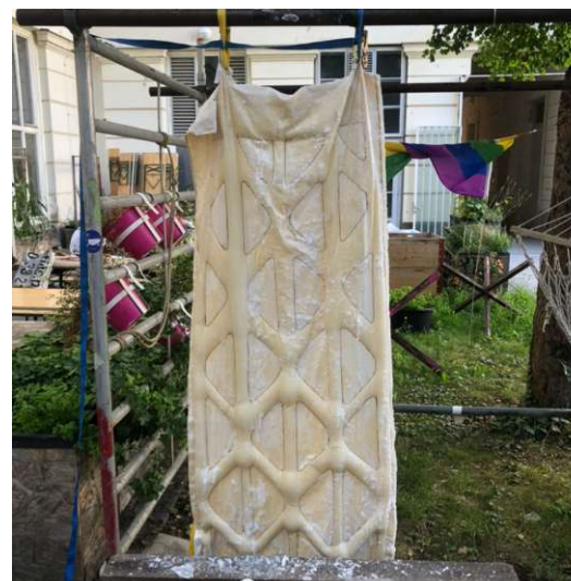
Fig. 188. The structure about half filled
