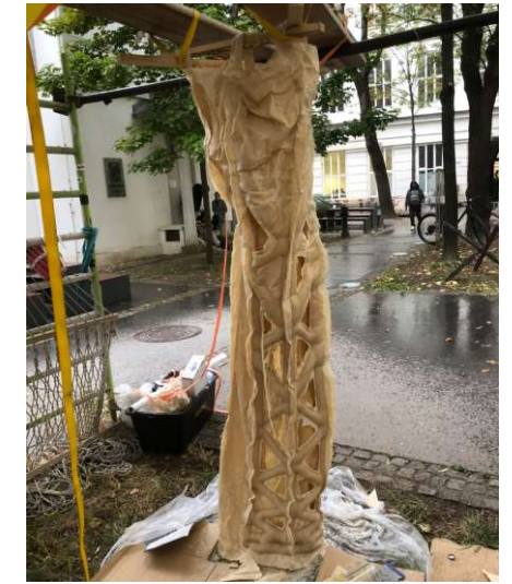
Fig.274. The formwork mostly filled
