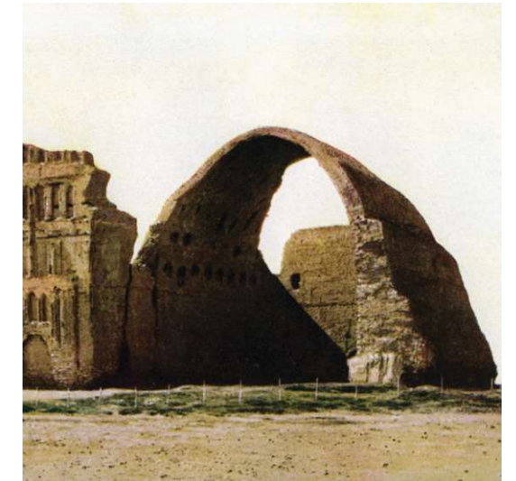
Fig.4. The Taq-I Kisra in Ctesiphon, Iraq an example of a catenary arc ca. 250-500 AD
