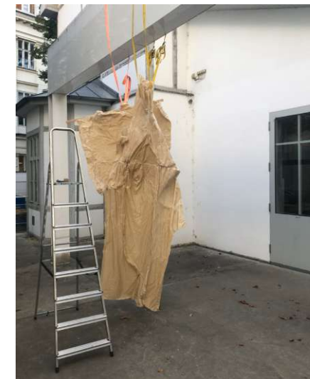
Fig.235. The formwork was hung on from a beam
