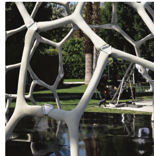
Fig.45. Steel triangles connect the modules
