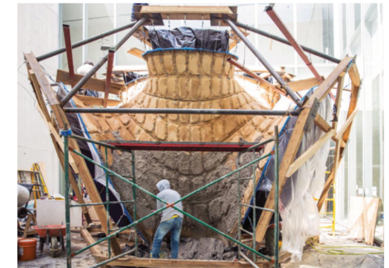
Fig.28. The temporary scaffolding
