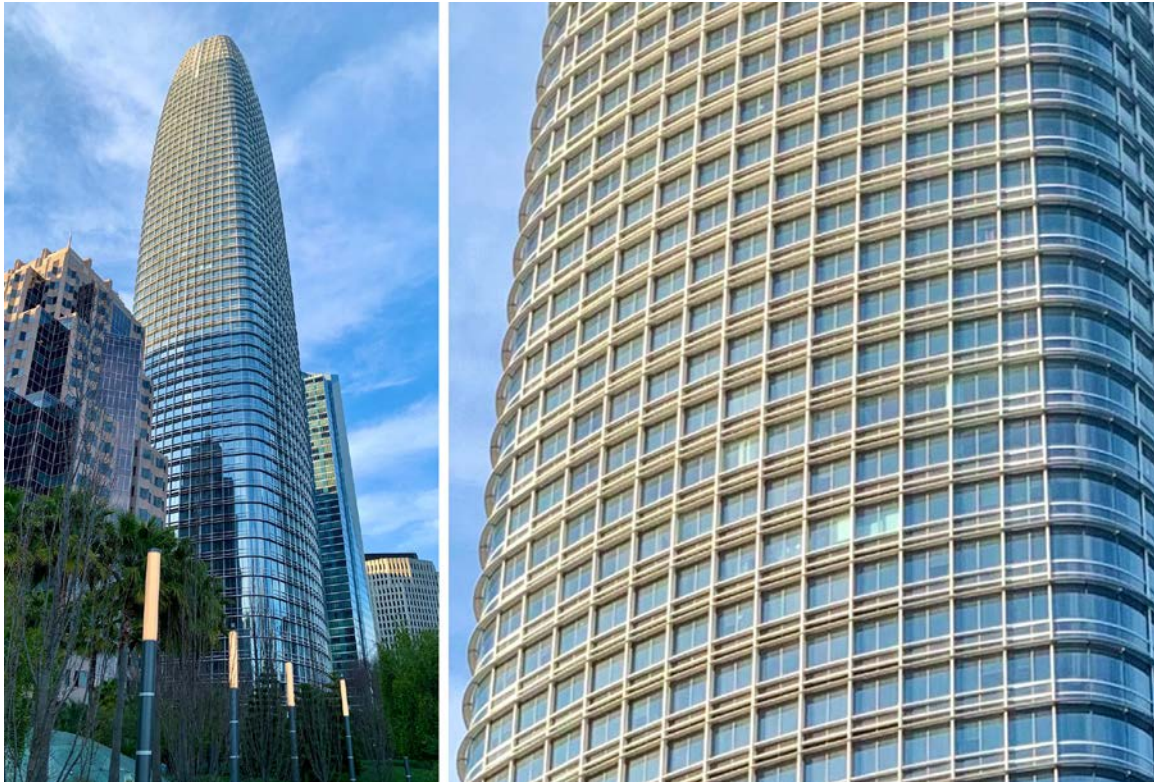
Figure 21. The Salesforce Tower, San Francisco, USA, completed in 2018, designed by César Pelli. Horizontal brise soleils above each floor and vertical fins on the facades deflect sunlight and provide shade. Source/Credit (©): photograph by Dead.rabbit via Wikimedia, licensed under CC BY-SA 4.0 [127] (right: cropped).
