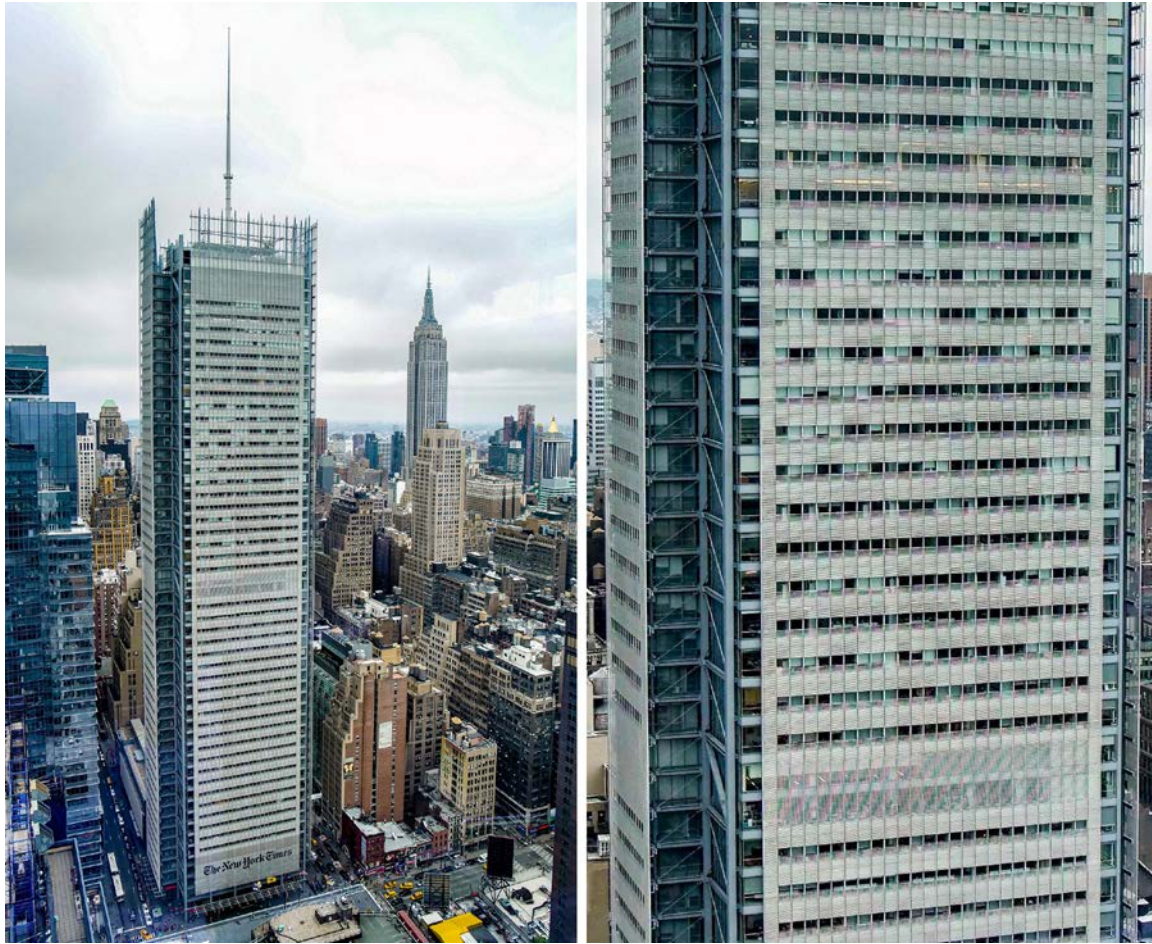
Figure 19. The New York Times Building (NYC, completed in 2007, designed by Renzo Piano and Fox & Fowle Architects) incorporated a DSF as a passive strategy to control the daylight and solar heat gain. Source/Credit (©): photograph by Defears via Wikimedia, licensed under CC BY-SA 4.0 [107] (right: cropped).
