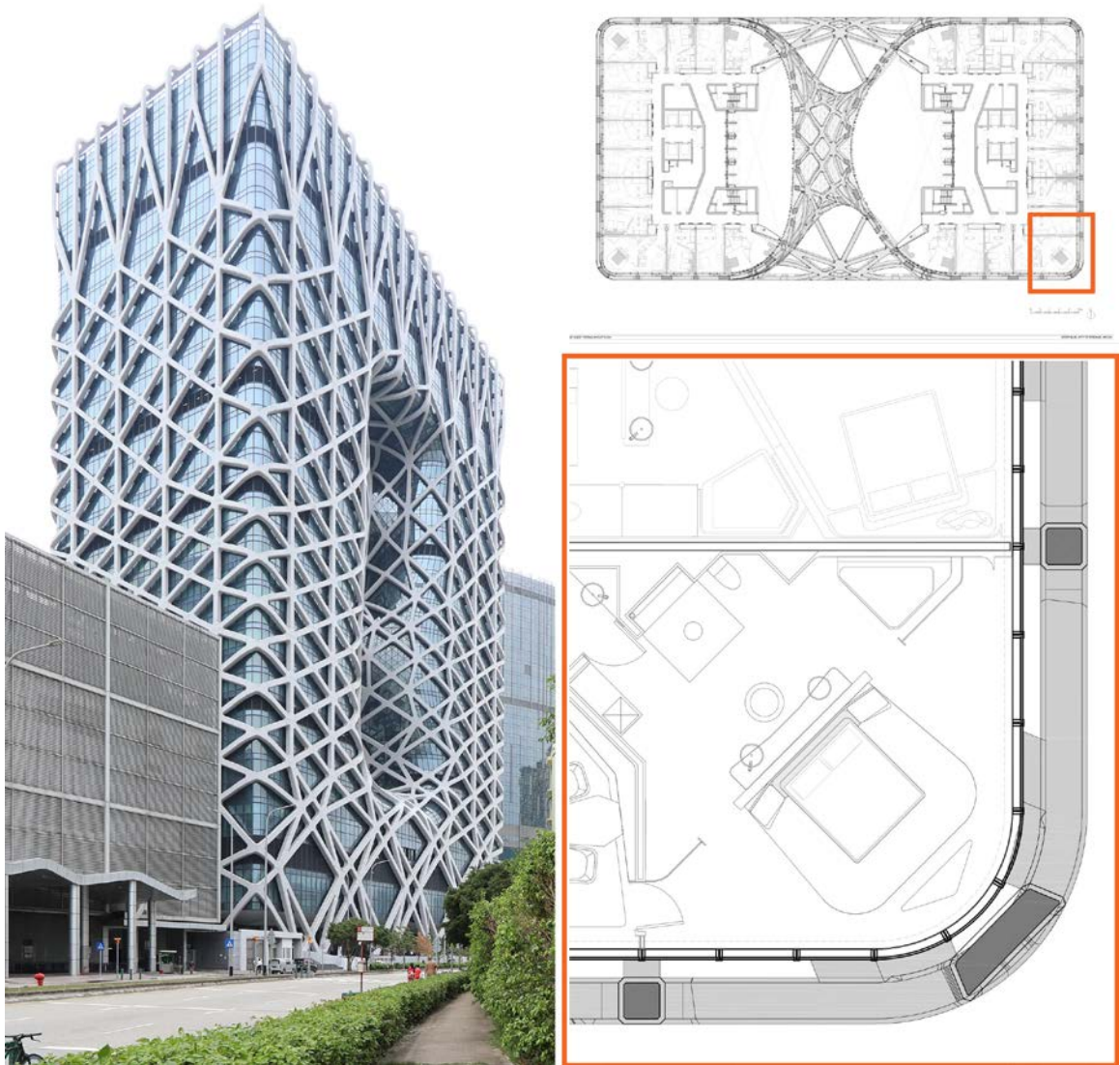
Figure 50. Example of the OUT level of the PTC factor; Morpheus Hotel by ZHA incorporates an exoskeleton diagrid frame that is fully placed in the exterior environment. Beams connect the exoskeleton to the rest of the structural system in the interior space. Sources/Credits (©): photograph by Störfix via Wikimedia, licensed under CC BY-SA 3.0 DE [18], cropped; drawing (25 th floor plan) courtesy of ZHA.
