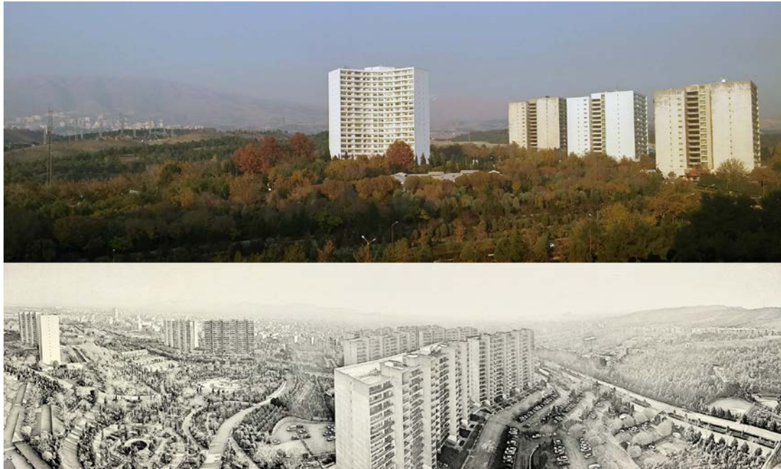
Figure 55. Shahrak-e-Omid, a residential neighborhood in Tehran, Iran, is noted for its relatively smaller built-up area and larger green spaces, which is a rarity compared to typical neighborhoods in Tehran. Source: photographs by the researcher
