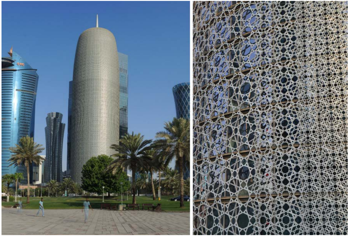
Figure 20. The Doha Tower (aka Burj Doha), Qatar, completed in 2012, designed by Jean Nouvel. The exterior skin of the DSFs constructed of multi-layered patterns invoking traditional screens designed to shade buildings from the sun, and protect the glass from sand residue. Sources/Credits (©): photographs, from left to right, by Axel Drainville [125] (cropped), and marc.desbordes [126], respectively, both via Flickr and licensed under CC BY-NC 2.0.
