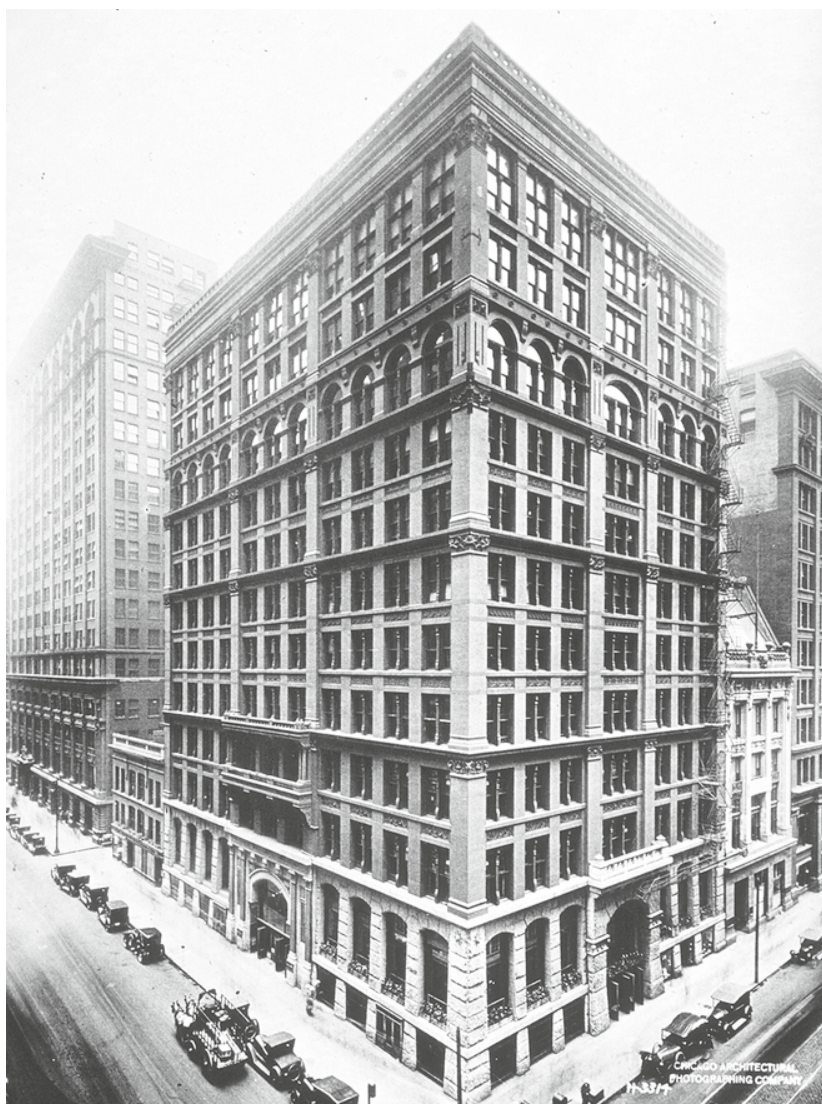
Figure 10. Home Insurance Building, Chicago, USA, completed in 1885, demolished in 1931, designed by William Le Baron Jenney, often considered the world's first modern tall building due to its pioneering use of iron frame skeleton with that height. Source/Credit (©): photograph by Chicago Architectural Photographing Company via Wikimedia, licensed under Public Domain [90].
