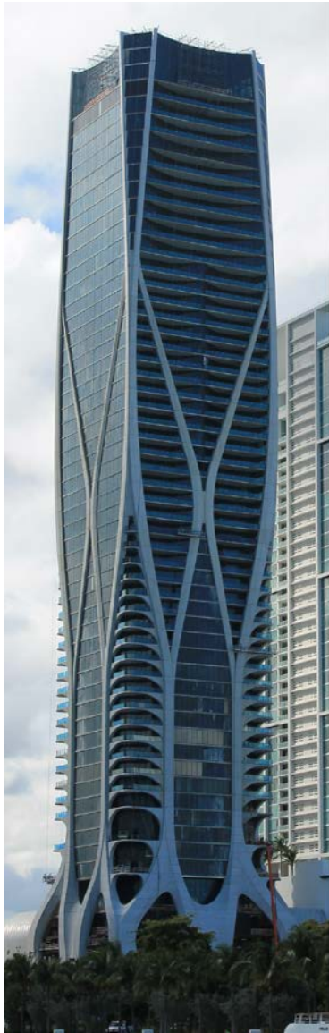
Figure 49. Example of the MID level of the PTC factor; One Thousand Museum, a high-rise residential building designed by ZHA, incorporates an exoskeleton in parts of which the (inclined) columns are centered with respect to the thermal envelope. For example, in the 28 th floor plan shown here, the columns on the top and bottom sides are partially in the interior space and partially exposed to the exterior environment. Sources/Credits (©): photograph by Godsfriendchuck via Wikimedia, licensed under CC BY-SA 4.0 [179], cropped; Floor plan, courtesy of ZHA.
