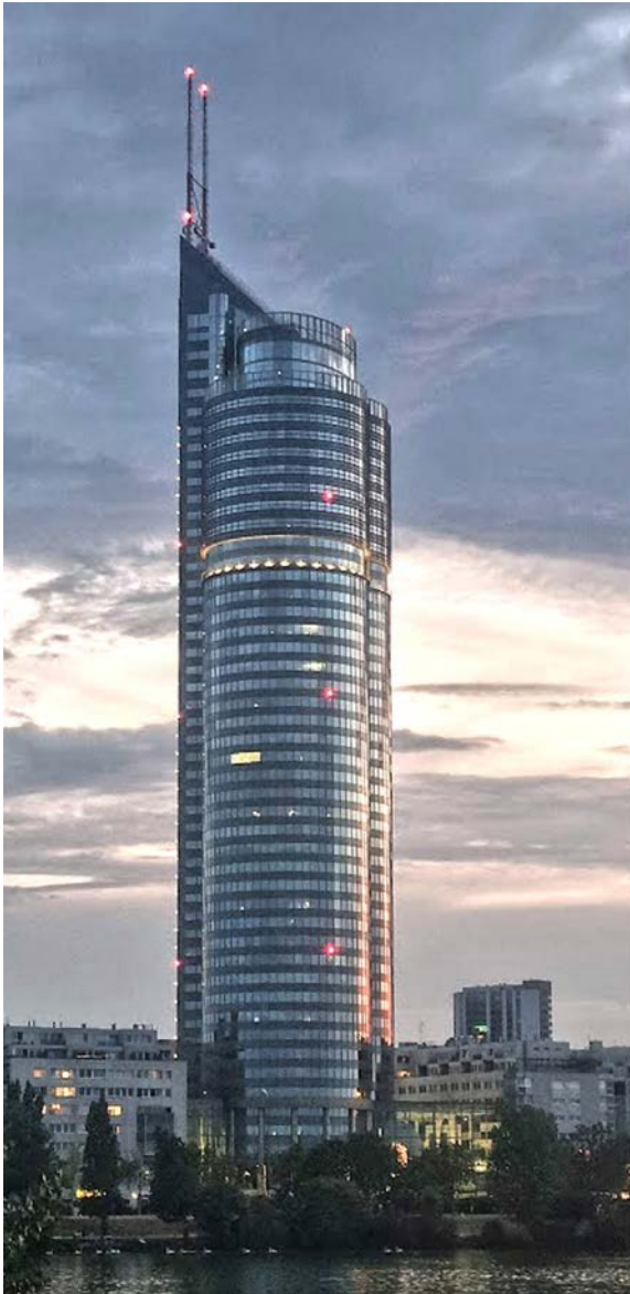
Figure 15. Ribbons of opaque panels separate ribbons of transparent glass windows in curtain wall facades of a contemporary tall building; Millennium Tower, Vienna, completed in 1999, designed by Gustav Peichl, Boris Podrecca and Rudolf Weber. Source: photographs by the researcher
