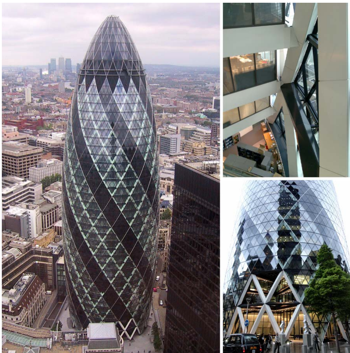
Figure 48. Example of the level IN of PTC factor; 30 St Mary Axe (formerly known as Swiss Re Building and commonly referred to as Gherkin), designed by Norman Foster, incorporates a diagrid frame as an endoskeleton. Although the skeleton is visible from the outside through the transparent portions of the facades, it remains almost entirely within the thermal envelope (see photos left and top right). There is only a relatively small part of the skeleton at the entrances that is directly exposed to the outside environment. Only these small parts can be considered exoskeletons (see bottom right photo). Sources/Credits (©): photographs by (left) BotMultichill and Elekhh via Wikimedia, licensed under Public Domain [176], cropped; (top right) Fastily via Wikimedia, licensed under CC BY-SA 3.0 [177]; (bottom right) Mark Hillary via Flickr, licensed under CC BY 2.0 [178].
