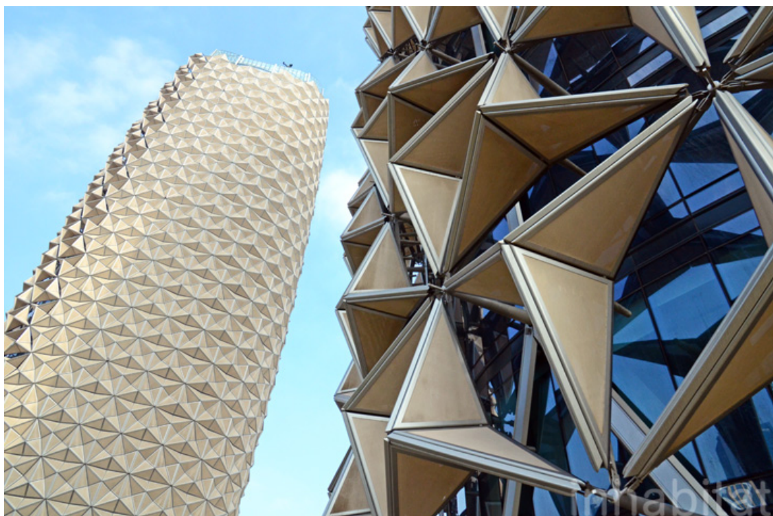
Figure 22. Al Bahr Towers (Abu Dhabi, UAE, completed in 2012, designed by AHR) feature an innovative active external shading system that comprises foldable modules that block glare and reduce heat gain and energy consumption while allowing indirect light to enter, promoting energy efficiency and user comfort. Source/Credit (©): photograph by Inhabitat via Flickr, licensed under CC BY-NC-ND 2.0 [129].
