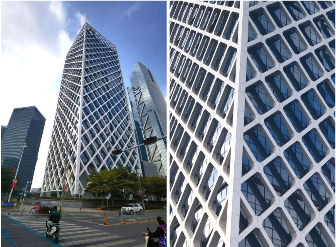
Figure 4. A tall building with a diagrid frame utilized as exoskeleton; Shenzhen Rural Commercial Bank Headquarters, Shenzhen, China, 2020, by SOM. Source/Credit (©): photograph by Lhzss8 via Wikimedia, licensed under CC BY-SA 4.0 [49] (brightness adjusted, right: cropped).
