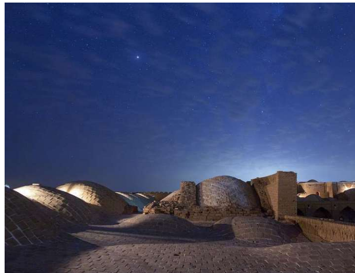
Abb1.20 : Qasr-e Bahram Karawansarei, begehbares Dach, Semnan, Iran
