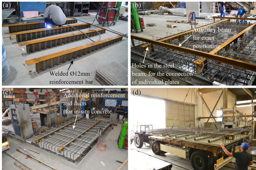
FIGURE 8 Construction of thin-walled prefabricated plates: (a) corrugated web steel girders with welded reinforcement; (b) reinforcement cage with steel girders, exactly positioned with an auxiliary beam; (c) concrete plate with attached steel girders and additional reinforcement and ducts; (d) finished concrete plate during lifting, before the transport
