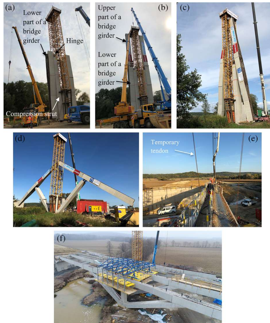
FIGURE 4 Construction steps of the Lahnbach bridge: (a) assembly of two compression struts and two lower parts of the bridge girders next to the pier; (b) assembly of the two upper parts of the bridge girder; (c) rotation initiation phase: Pushing the compression struts apart; (d) lowering process; (e) filling the U-shaped girders with pumped in situ concrete; (f) construction of the carriageway slab with a formwork carriage, taken from Ref. 9
