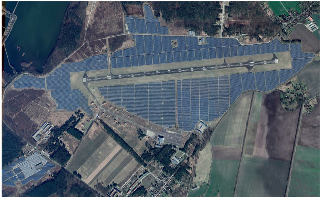
Fig. 3 Free-field photovoltaic plant with 145 MW p installed on an area of 240 ha in Neuhausen, Germany [14] (Google Earth, 2019 [13], image recording data: 3 February 2017)
