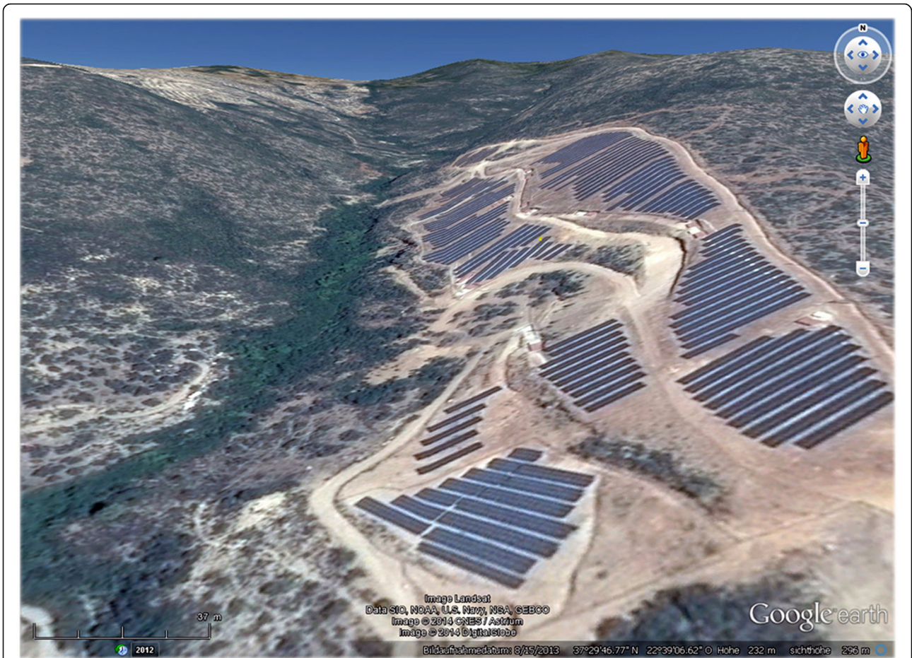
Fig. 1 Free-field photovoltaic plant with an installed power of 3 MW p in the mountains near Velanidia, Peloponnese region, Greece (Google Earth, 2019 [13], image recording data: 26 October 2013)
