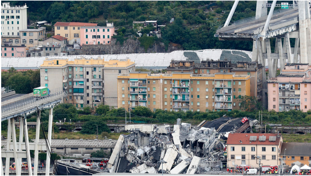
Fig. 1.1: On the 14th of August 2018 the motorway bridge "Ponte Morandi" in Genoa, Italy, collapsed (from http://press24.net )
