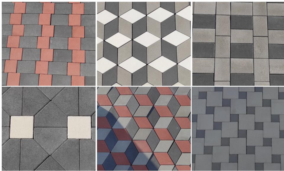
Fig. 2. 1. Concrete paving stone laying pattern [11]
