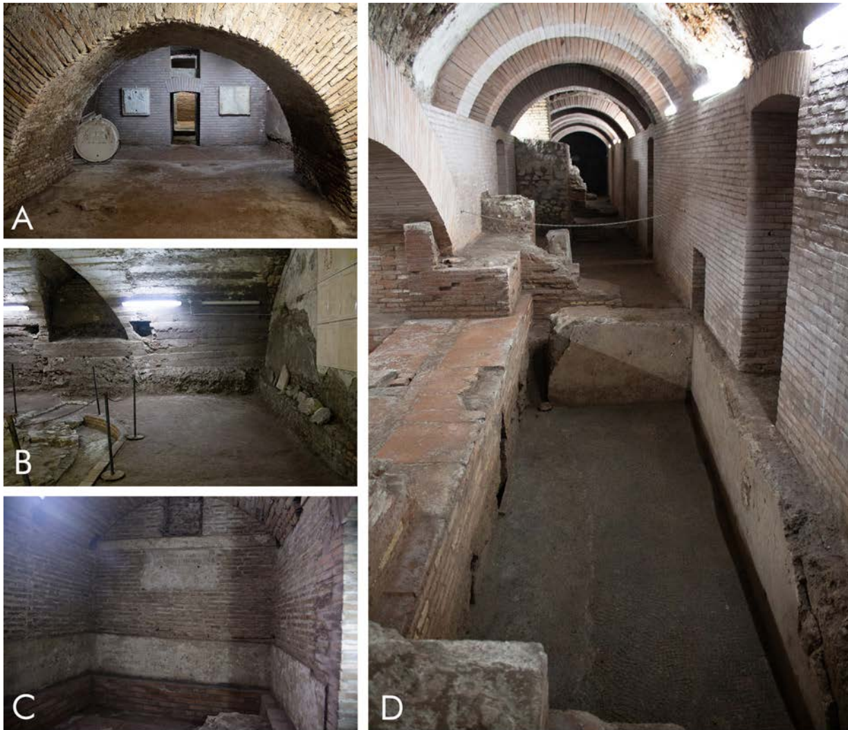
Figure 4. Some accessible rooms in the basement of the Basilica.
