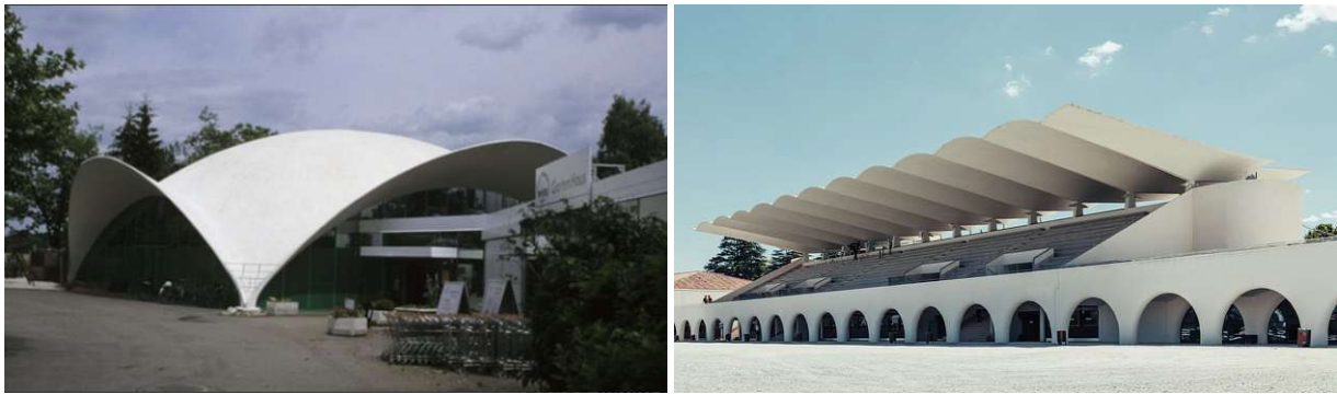
(a) Wyss Garden Center, Solothurn, 1961 Quelle: https://structurae.net/en/structures/wyss-garden-center
