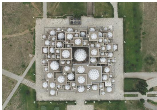
Figure 1 - Aerial view of the library (Kosovo Architecture Foundation 2018)
