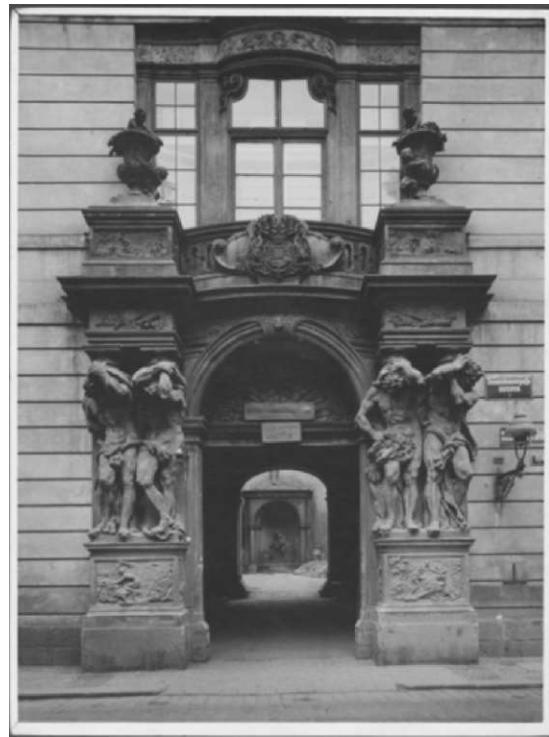
Img 5.23: Clam-Gallas Palace - Right Gate 1945 (Prague Archive)
