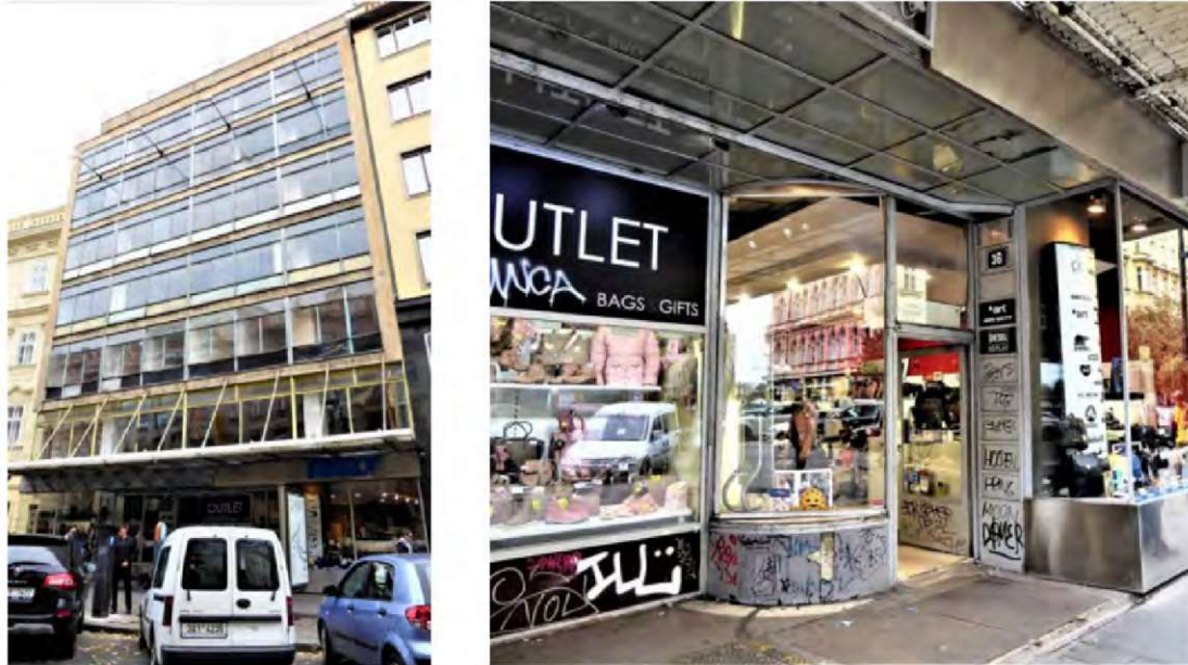
Img 5.12: Design Palace current situation (Design Cabinet)
