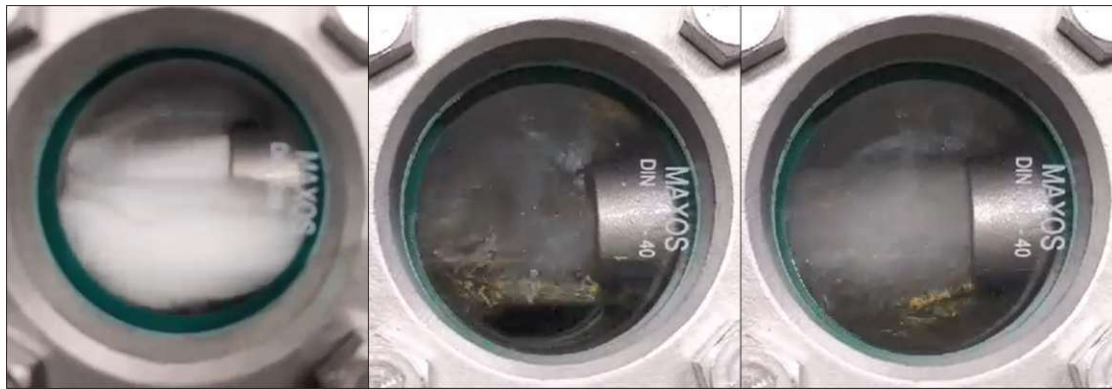
Figure 36: Although the pressures and temperatures mostly indicated subcooling at the motive nozzle of the ejector, in the sight glass upstream of the motive nozzle turbulent two-phase flow was visible. (Pictures taken by OCH and the author.)
