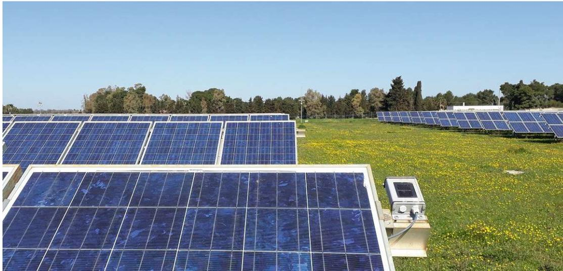
Figure 2.3: Photovoltaic panels and a silicon sensor installed in the Plane of Array (POA). Image credit: [34]
