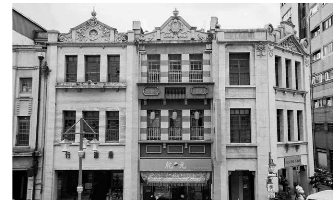
Fig.5 Modern architectural street house
