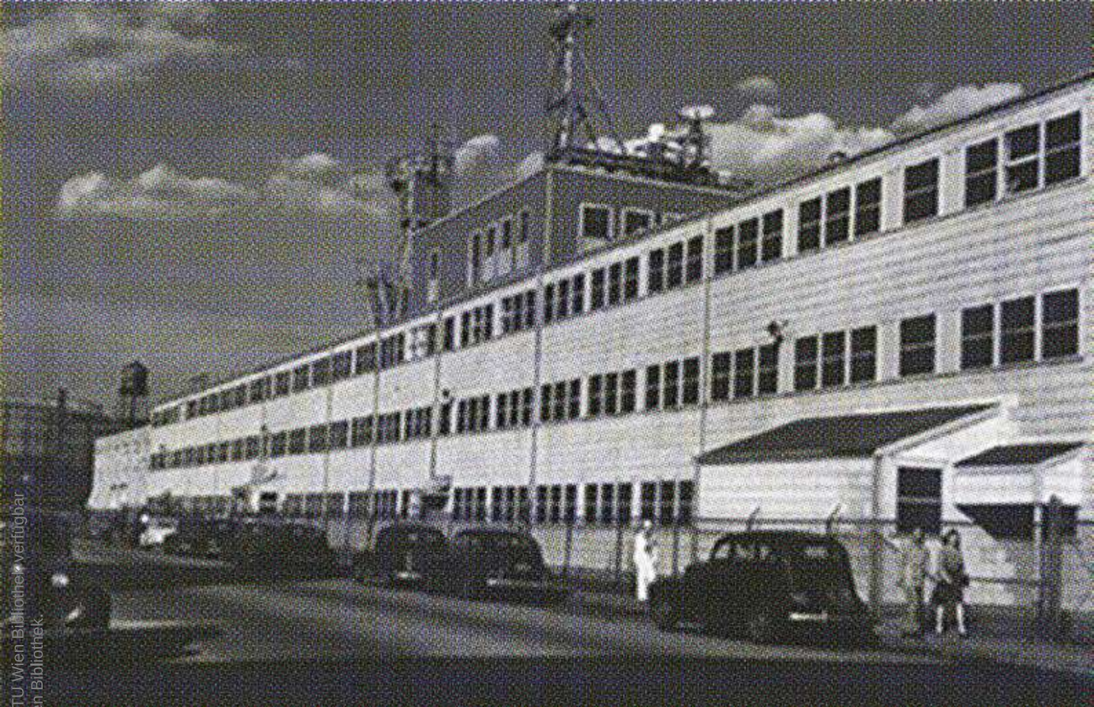
Figure 13: Building 20, 18 Vassar Street in Cambridge, Boston
