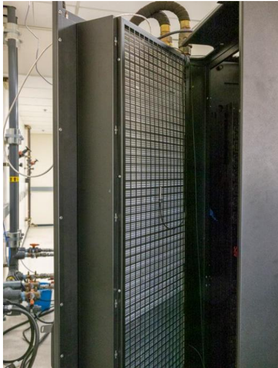
Fig. 12 shows the typical liquid cooling rear door heat exchanger (Loyolan Ventures, 2021)
