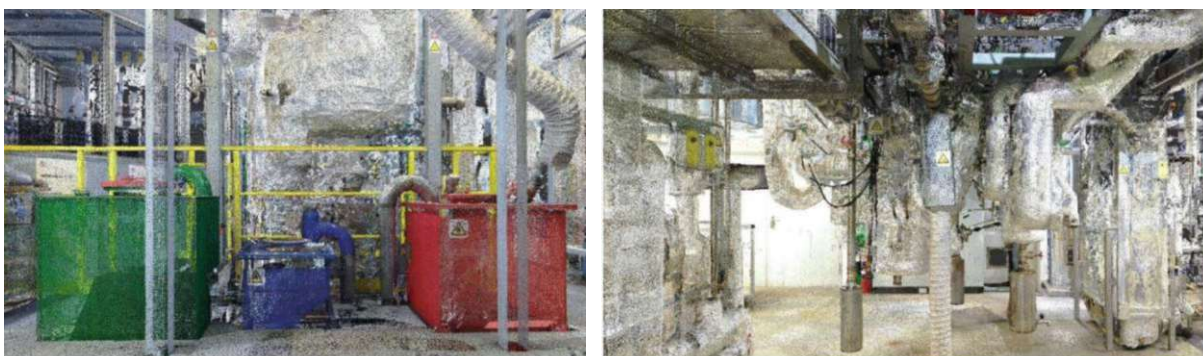
Figure 65: Pictures of a 3D scan of the gasification test plant at TU Wien
