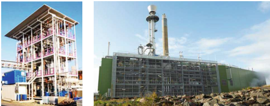
Figure 50: A 1 MW demonstration plant, Güssing [TRL 5] (left); a 32 MW Plant, Goteborg [TRL 7] (right)
