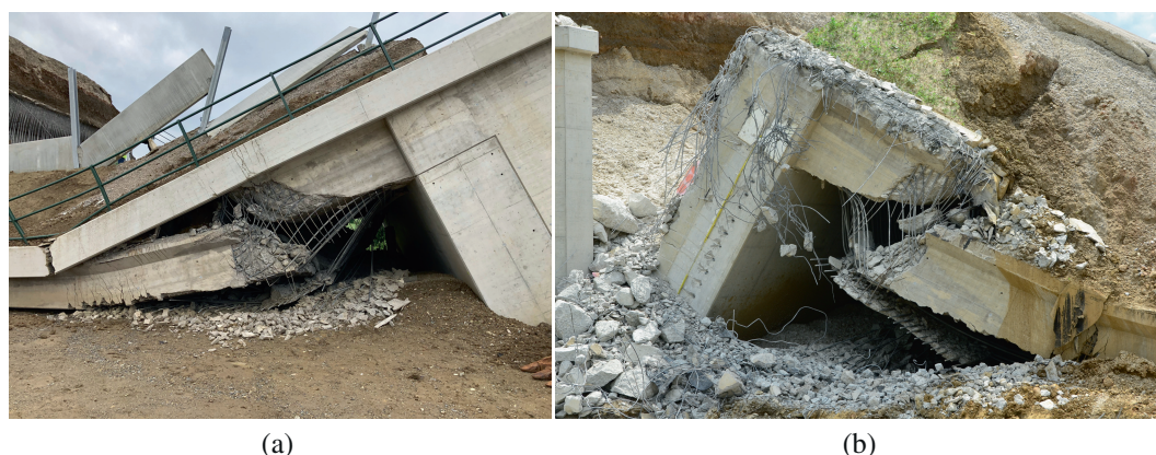
FIGURE 5 Tilted abutment 20 with shear crack: (a) from the south-west; (b) from the north-east.
