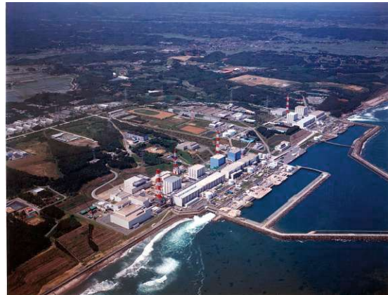
(b) Photo of the FDNPP site in February 2007. Source: [2]
