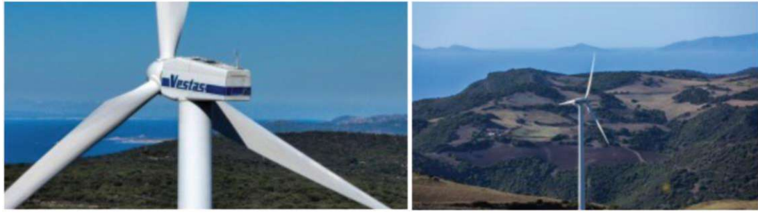
Figure 28 - Wind turbine Vestas V52 18
