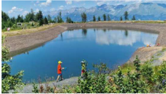
Figure 46 - 75000 m 3 reservoir, partly empty
