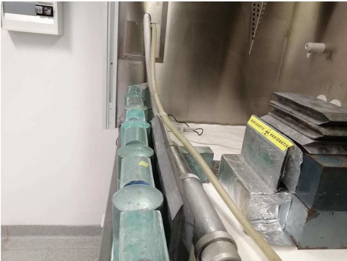
Figure 6 Entrance and starting point of the pneumatic transfer system.
