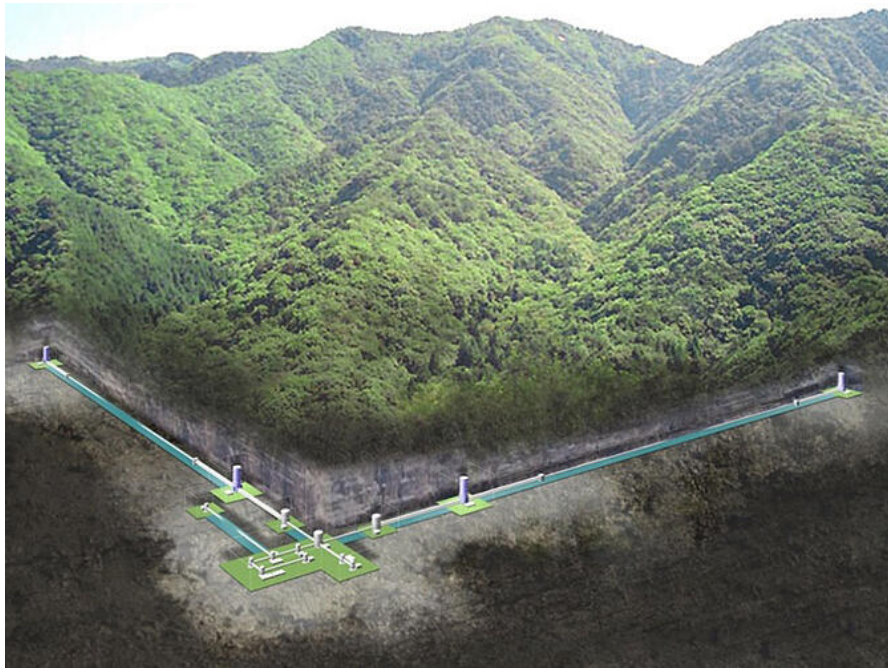
Figure 3.4.: Overhead view of the underground KAGRA gravitational wave observatory, featuring 3 km-long arms forming an L-shaped tunnel [40].
