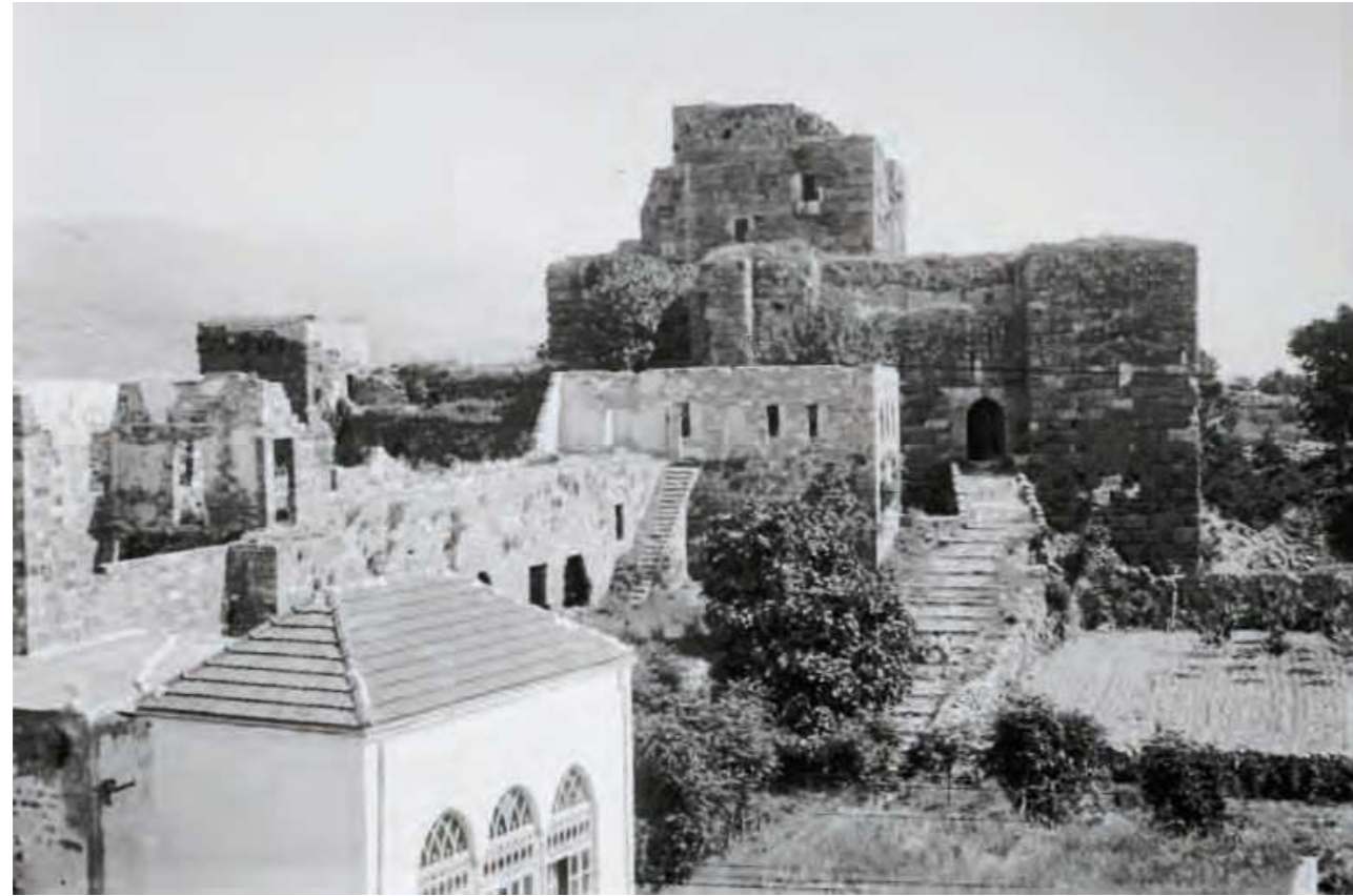
Fig 46. Northern facade. Lebanon Archive, 1926.
