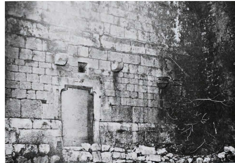
Fig 45. External doorway. Camille Enlart, 1921.
