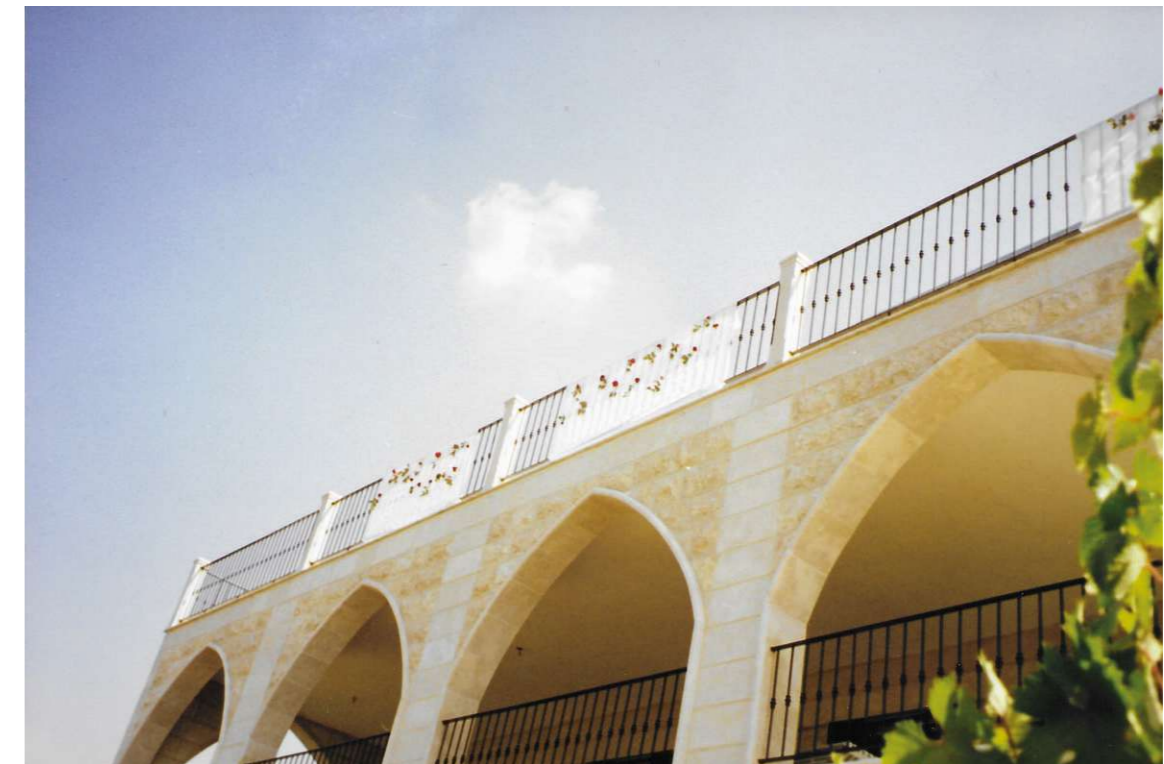
Fig 91. Facade of the upper floors. Bejjeh, Mount Lebanon. 2003.
