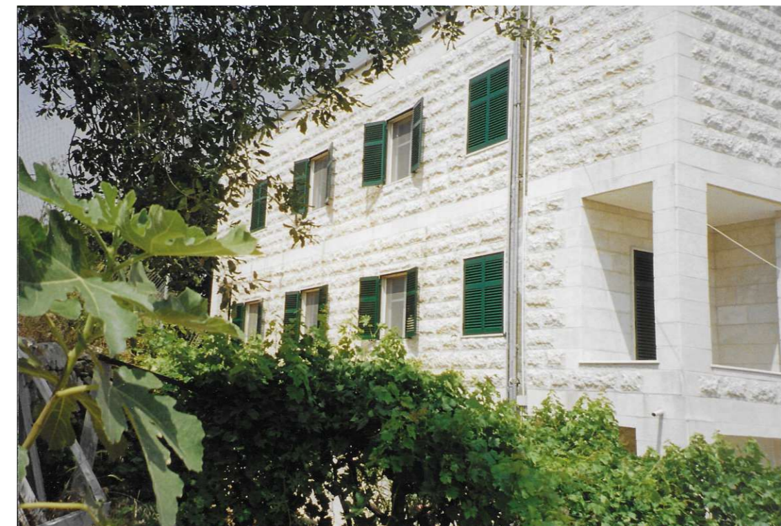
Fig 85. South-eastern facade. Bejjeh, Mount Lebanon. 2004.
