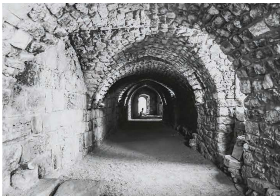
Fig 50. Passageway by the yard. Moovtoo, 2023.
