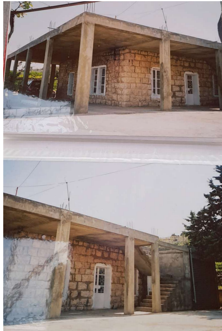
Fig 80. The original house, built in 1947, with reinforced concrete posts (60s) and a staircase (80s) added later. Bejjeh, Mount Lebanon. 1992.
