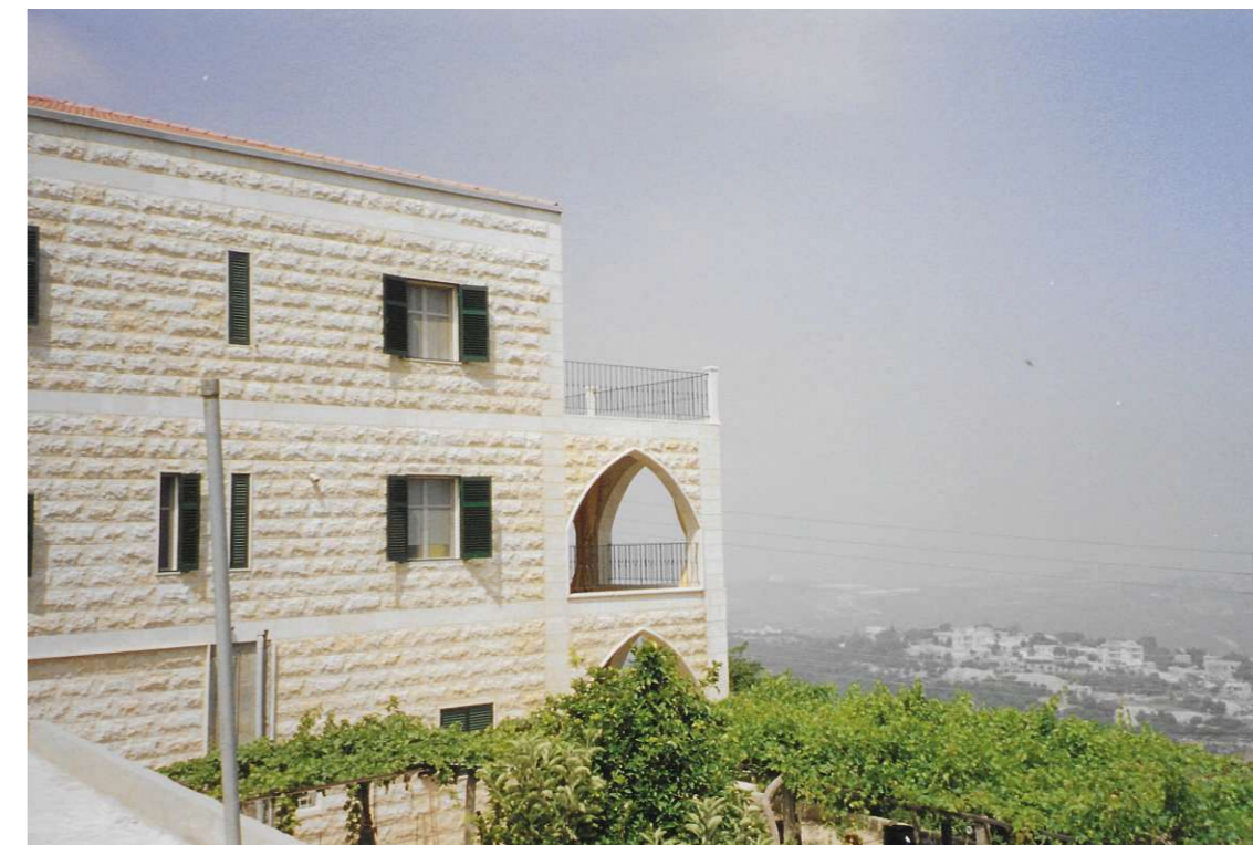
Fig 84. North-eastern facade. Bejjeh, Mount Lebanon. 2004.
