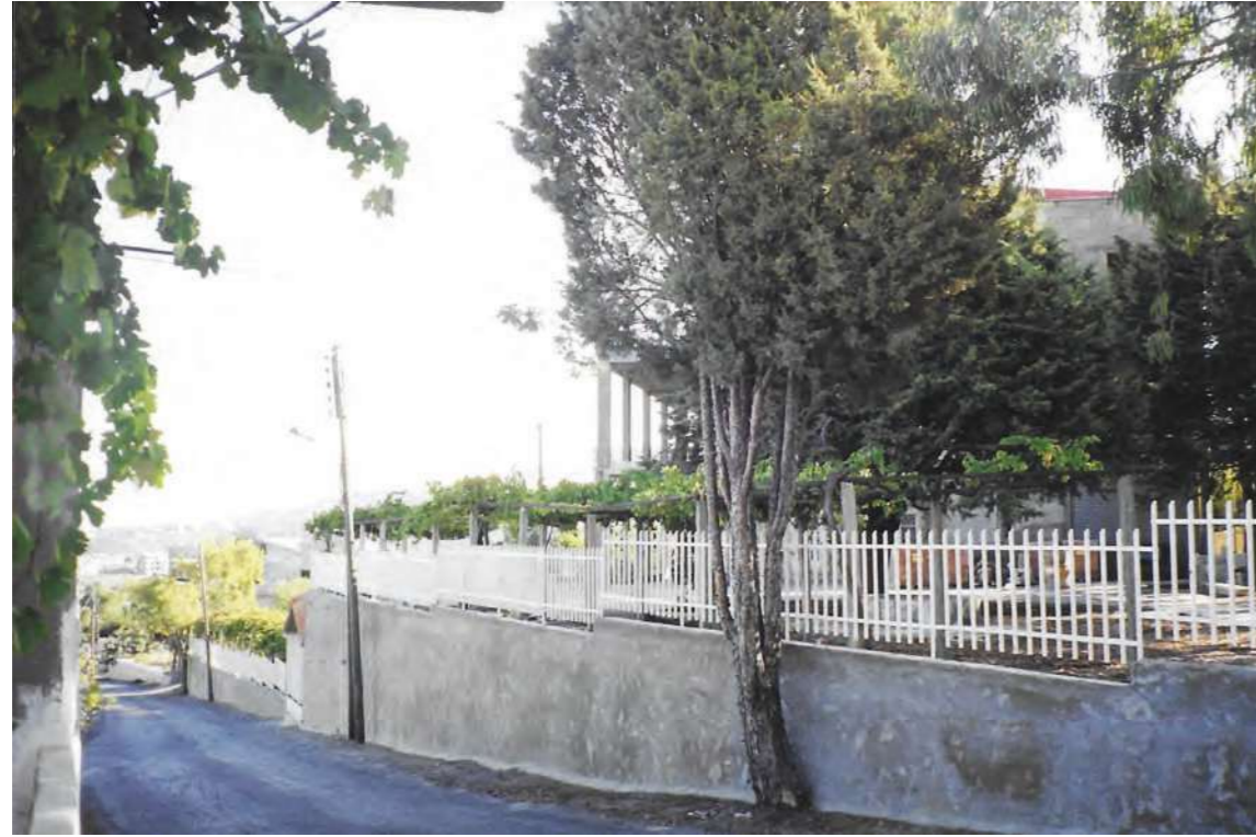
Fig 92. Main road and retaining wall. Bejjeh, Mount Lebanon. 1992.
