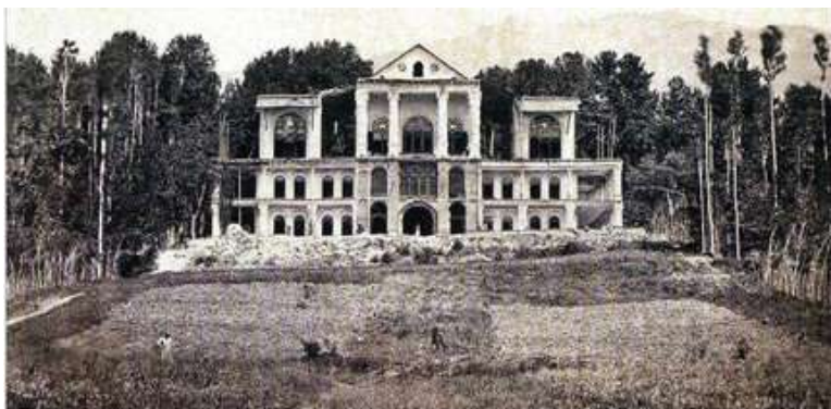
Figure 68. Ferdows Garden's mansion in 1879 as a Qajar mansion in Tajrish, south of Darband
