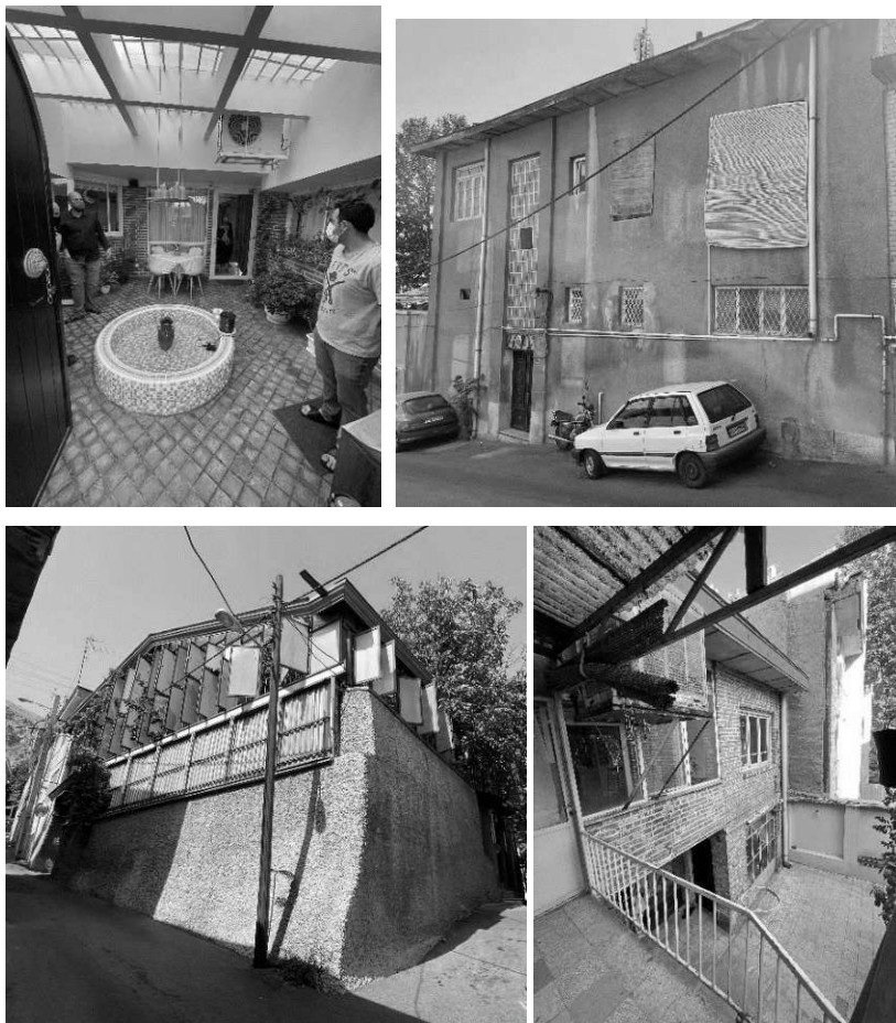
Figure 161. Alteration in the current houses of Darband to achieve privacy
