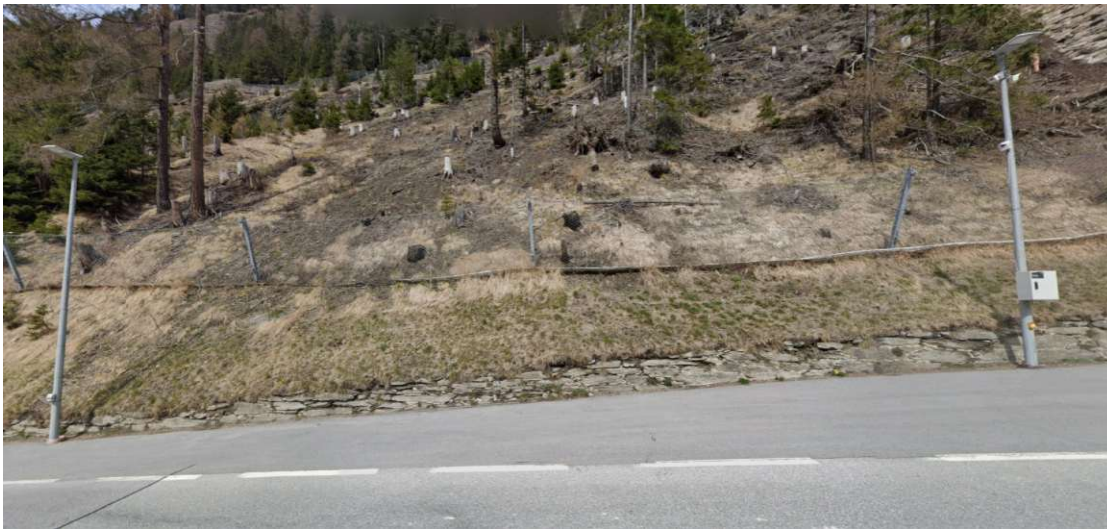
Figure 5.2: Camera and sensorbox setup at B182 Brennerstraße
