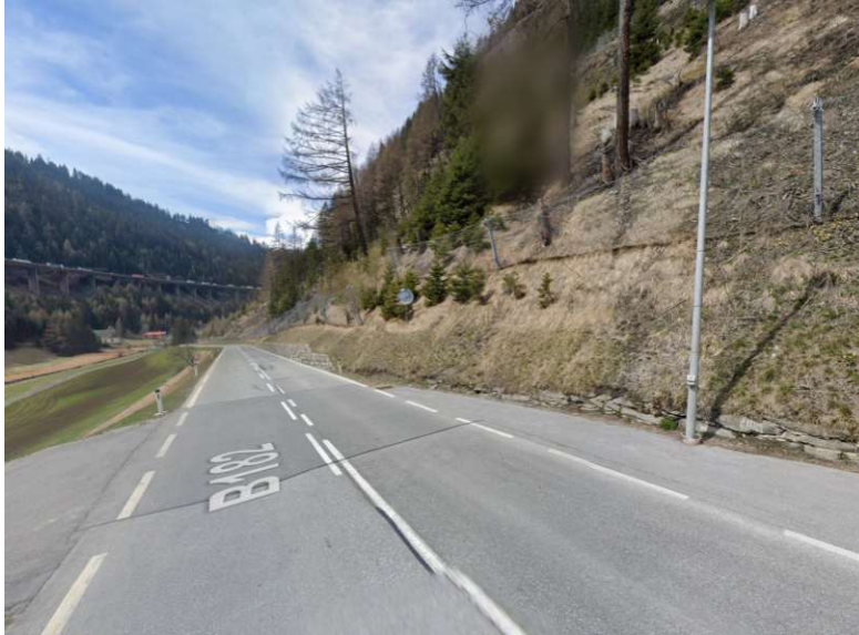
Figure 5.1: Sensor box setup at B182 Brennerstraße
