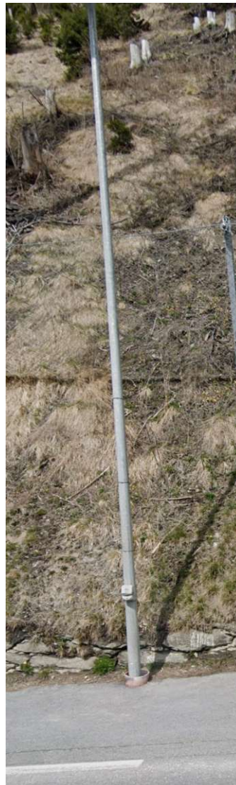
Figure 5.4: Sensor box setup at B182 Brennerstraße
