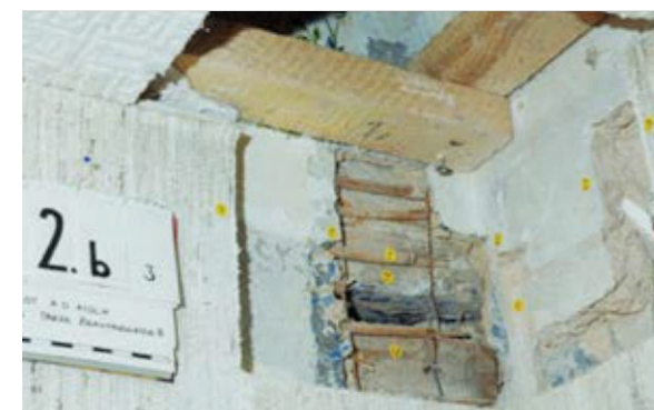
13 | Examination of Wall and Ceiling Layers
