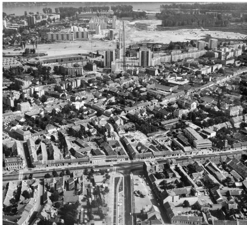
Fig 6. Construction of 23rd October Boulevard (now Boulevard of Liberation)
