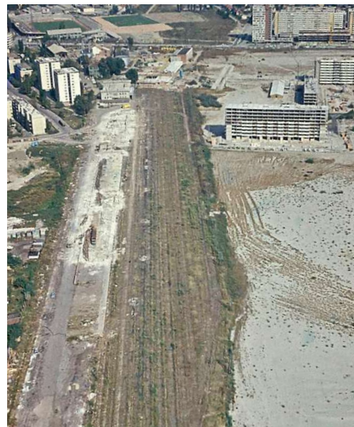
Fig 7. Removal of the Old Railway Station, 1970
