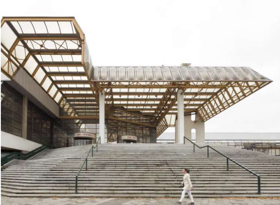
Fig 17. North Entrance Platform
