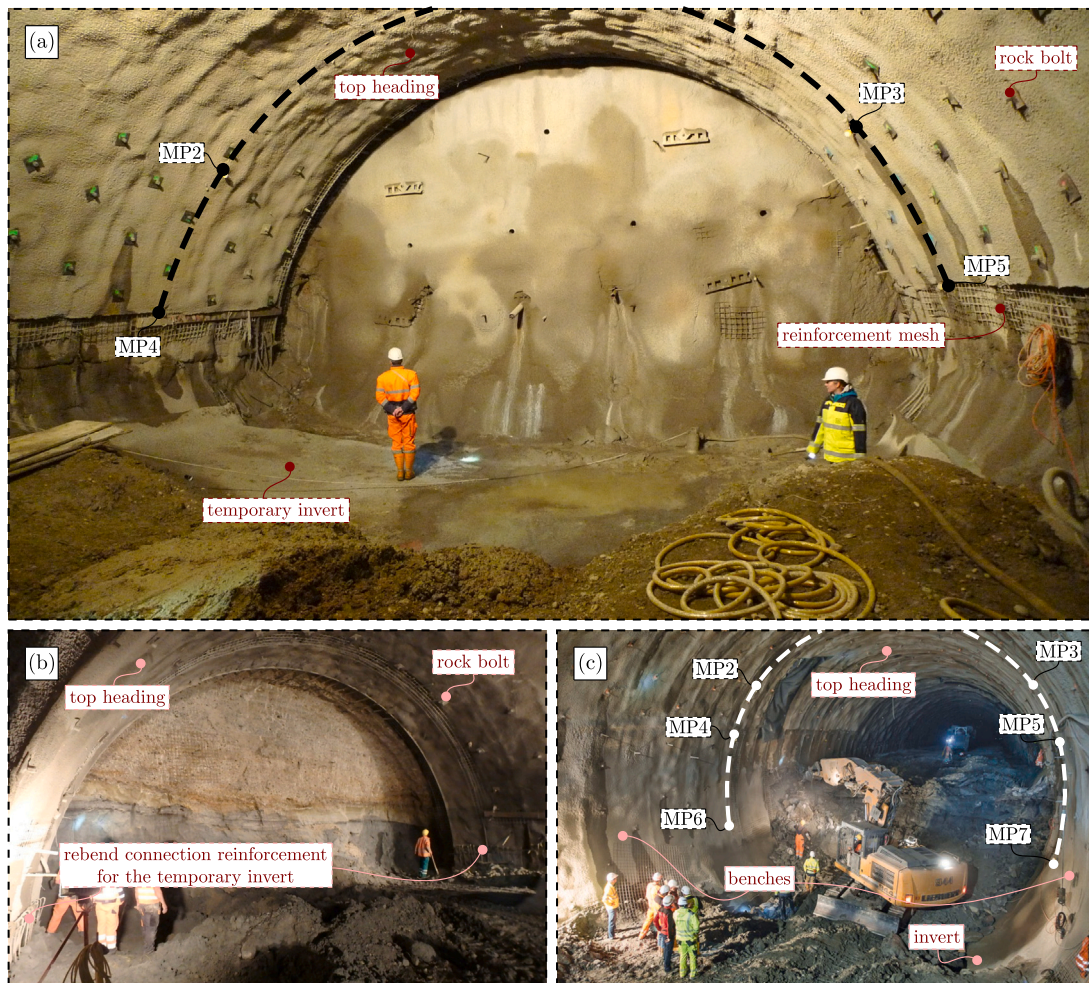
Fig. 4. Construction and monitoring photos of tunnel Stein: (a) top heading and temporary invert installed, (b) installation of top heading only, and (c) excavation of the benches; with labeling of tunnel shell portions, rock bolts, reinforcement elements, and measurement point locations, photographs (a) and (b) by courtesy of ÖBB-Infrastruktur AG; photograph (c) reproduced from Figure 6 of (Herzeg and Moraus, 2017), with permission of John Wiley and Sons.
