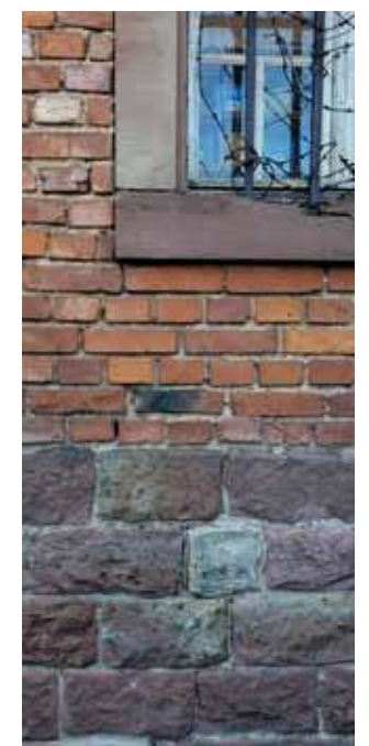
Abb. 132 - Sockeldetail
