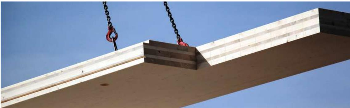
Abb.84: Brettsperrholz (BSP/CLT) Massivholzplatte
